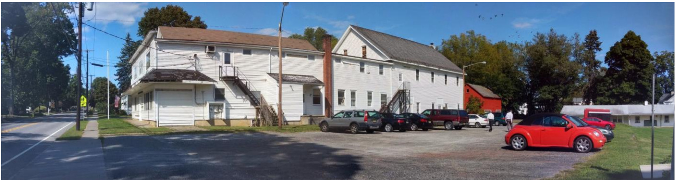
Southerly Side of Building and Lot
