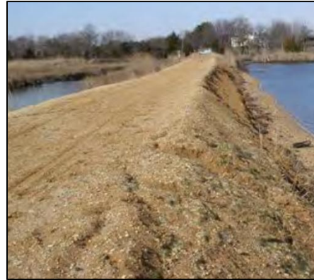
Figure 5.3-10. Cracking
