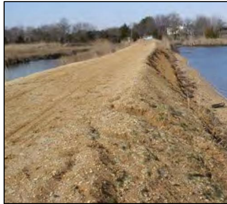
Figure 5.3-10. Cracking
