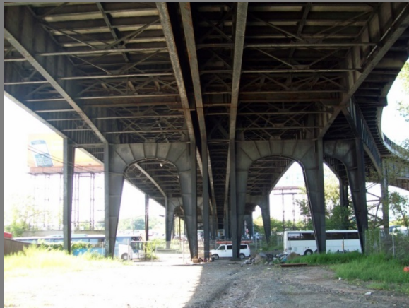
Complex Viaduct and Connected Ramp Framing
