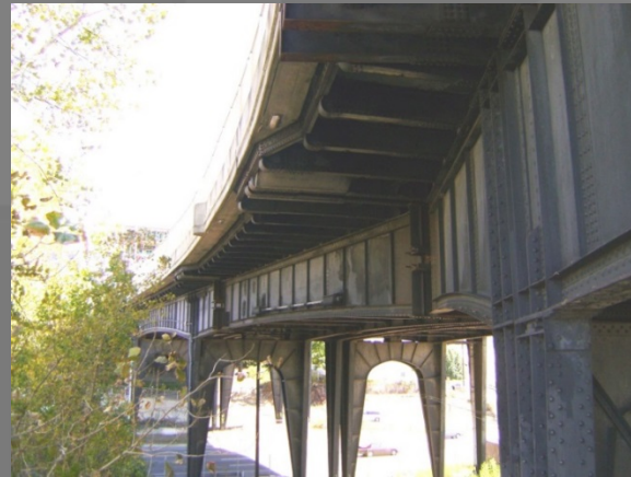
Complex Viaduct and Connected Ramp Framing
