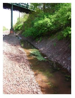
The NW quadrant contained a ditch with steady flow to the south. The ditch flowed into a plastic culvert approximately 20 feet north of the bridge support structure. The outflow of this culvert could not be located in the vicinity. This ditch contained no vegetation and also appeared to have been recently altered (both photos below: right is toward crossing and left is upstream/north). This ditch does not posses wetland characteristics but appears to constitute state open water.
