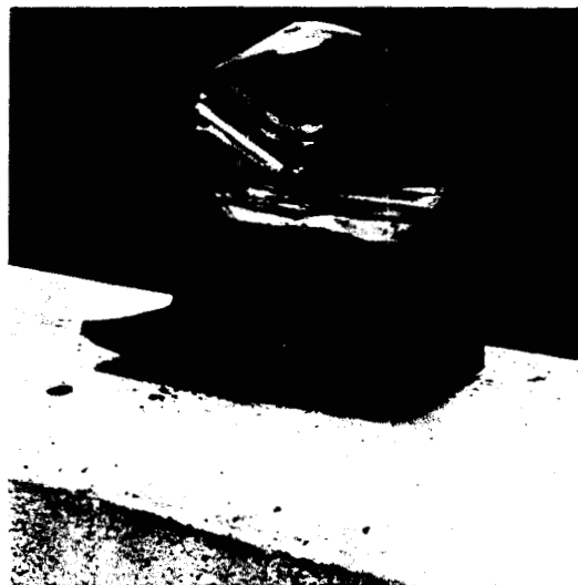
INSTALLED PERPENDICULAR TO INTENDED POSITION REFLECTORS NOT VISIBLE TO MOTORISTS
