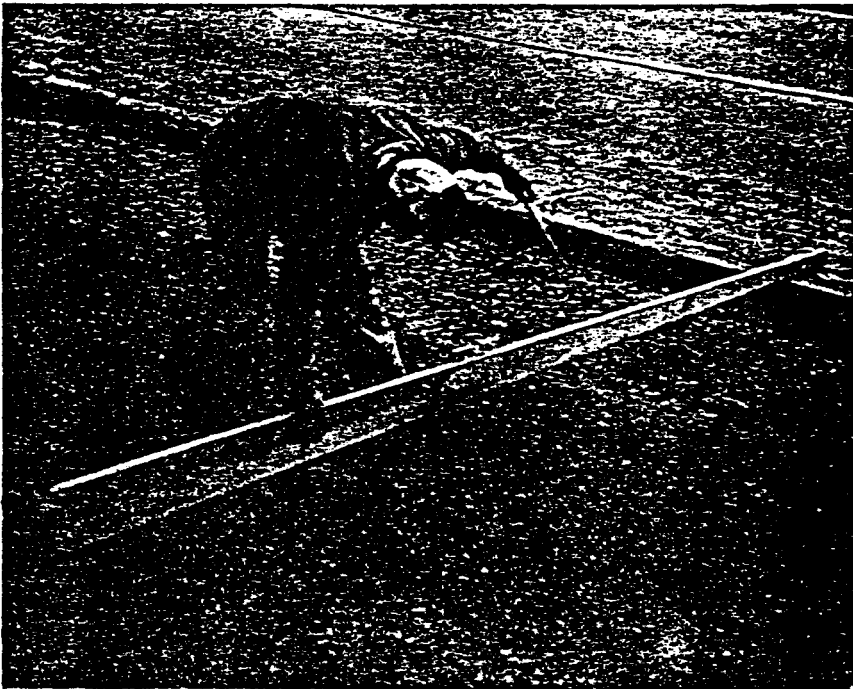
FIGURE 14 Checking Grade
