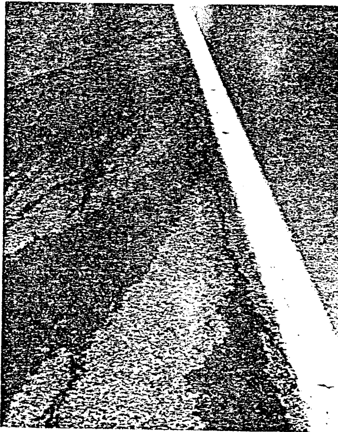
Figure 7: Route 287 southbound @ M.P. 31-1/2. Inadequate surface drainage can cause such a failure.
