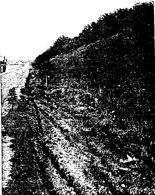
Figure 13: Route 78 eastbound @ M.P. 25-1/2. When no drainage is provided runoff makes provision on its own.
