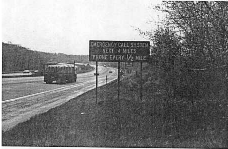
FIGURE 2 - I-80 SYSTEM'S ADVANCED SIGNING
