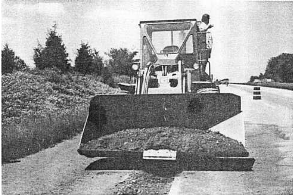
No. 9 - Excavation For Inlay of Lime-Fly Ash
