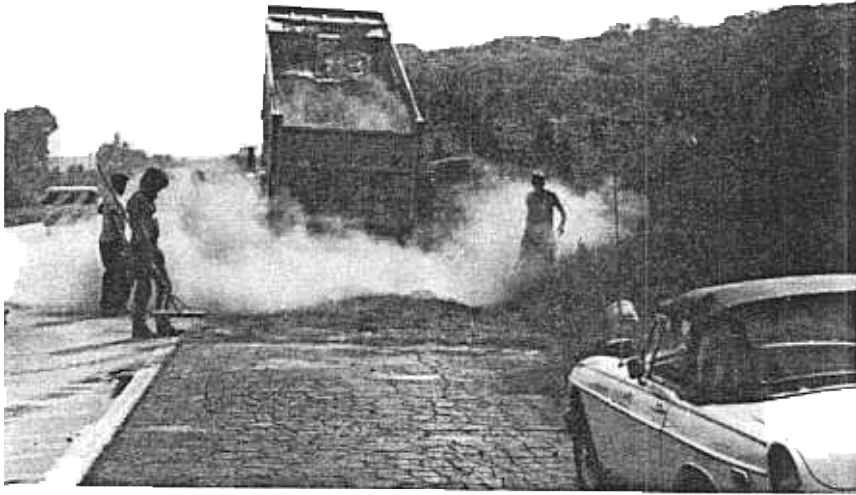
No. 1 - Tail Gate Unloading of Lime-Fly Ash
