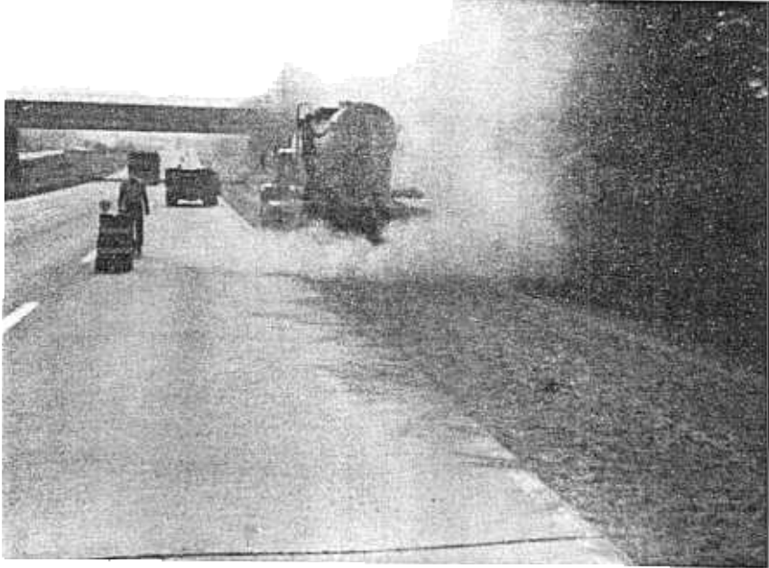
No. 5 - Pneumatic Placement of Cement
