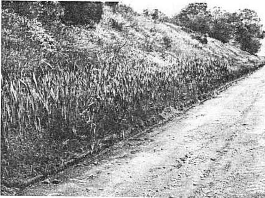
No. 13 - Install Drainage Ditches
