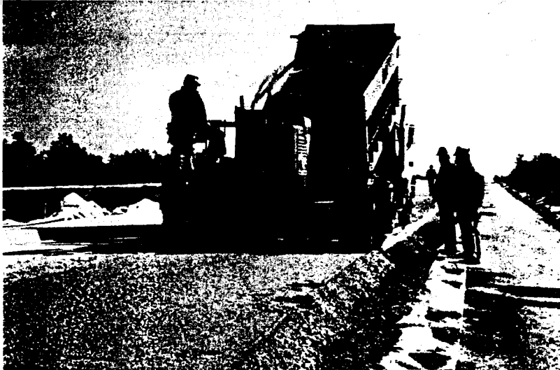
FIGURE 35. Route 195, Placing of the NSOG Layer by an Asphalt Paver
