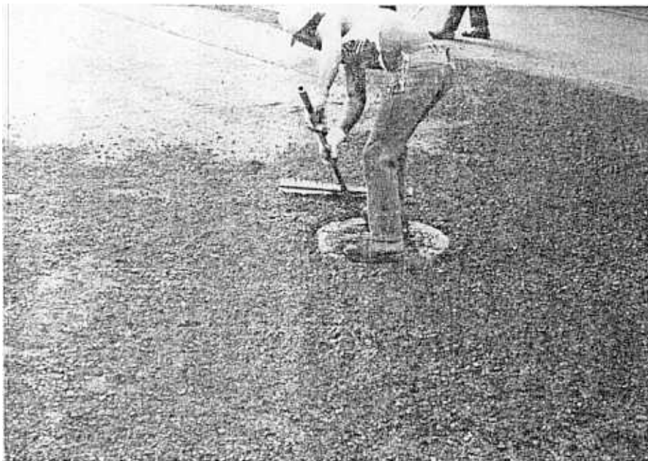
PHOTO 14 EXCESSIVE FEATHERING AND MIX SEGREGATION
