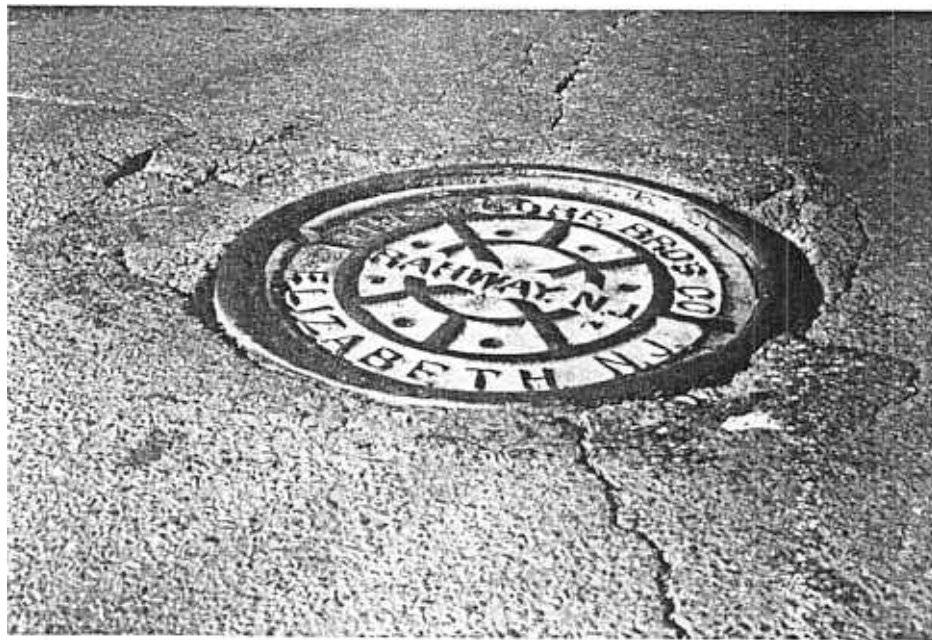
PHOTOS 5 & 6 (UNIFORM WEAR) COVER DEPRESSED DUE TO WEAR OF COVER SEAT
