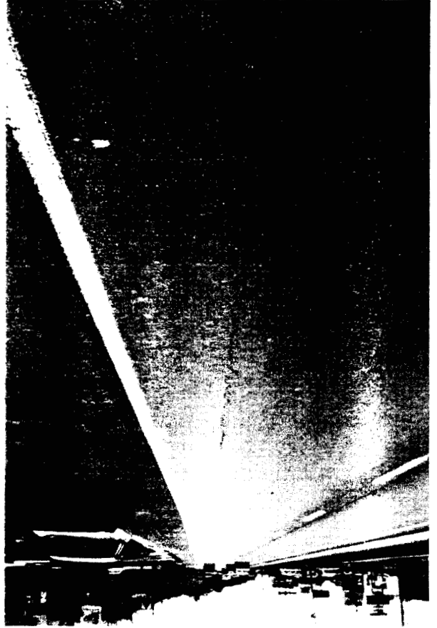
LONGITUDINAL SAW AND SEAL EDGE JOINT IN TEST SECTION
