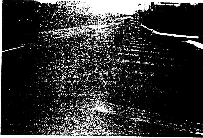
PHOTO 11 MILLING WITH NEW DRUM - NEW TEETH
