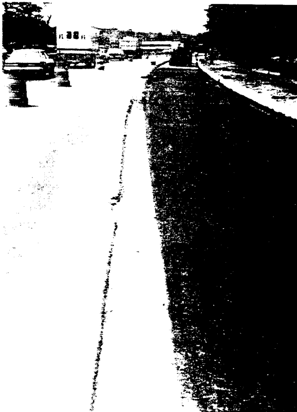
PHOTO 34 JAGGED EDGE CUT BACK OVER CONCRETE ON ROUTE 10
