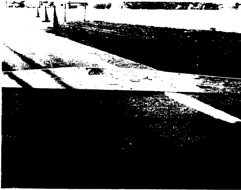
PHOTO 15 PAVEMENT CONDITION ON ROUTE 1 PROJECT PRIOR TO OVERLAY
