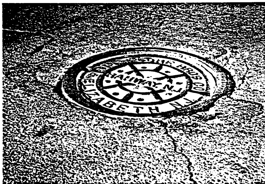
PHOTOS 5 & 6 (UNIFORM WEAR) COVER DEPRESSED DUE TO WEAR OF COVER SEAT
