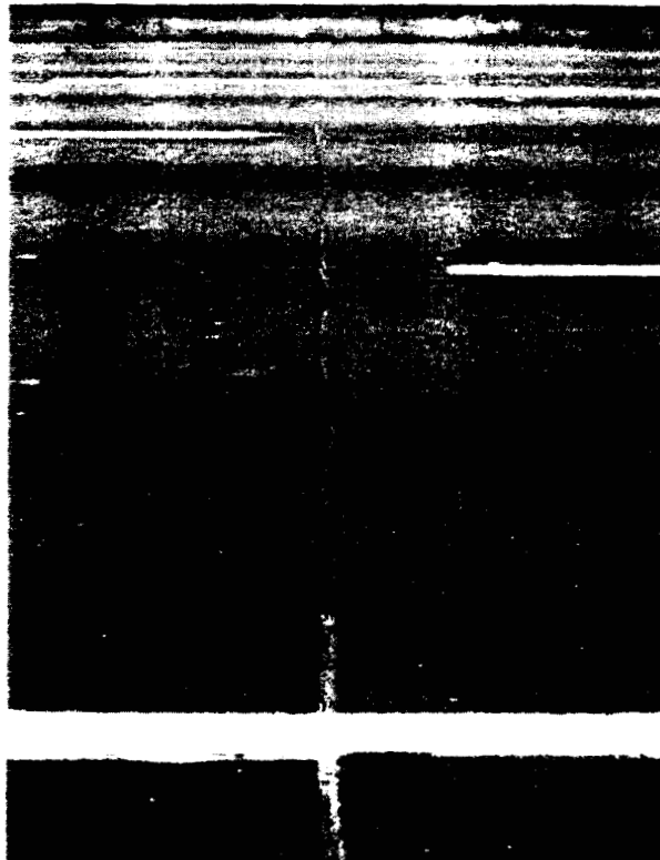
PHOTOS 60 & 61 REFLECTION CRACKING IN I-80 CONTROL SECTION
