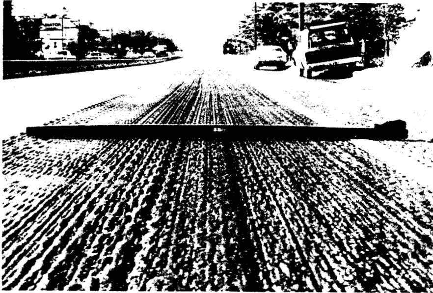
PHOTO 5 IMPROPER CROSS SLOPE DUE TO USE OF 2 MACHINES
