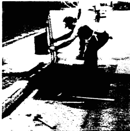
REPLACING GRATE
