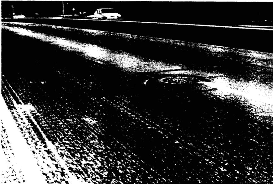
PHOTO 6 POOR WORKMANSHIP AT MANHOLE
