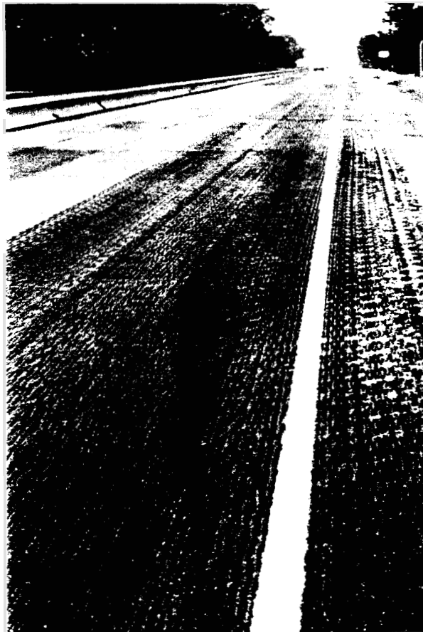
PHOTO 2 POOR MILLING TEXTURE
