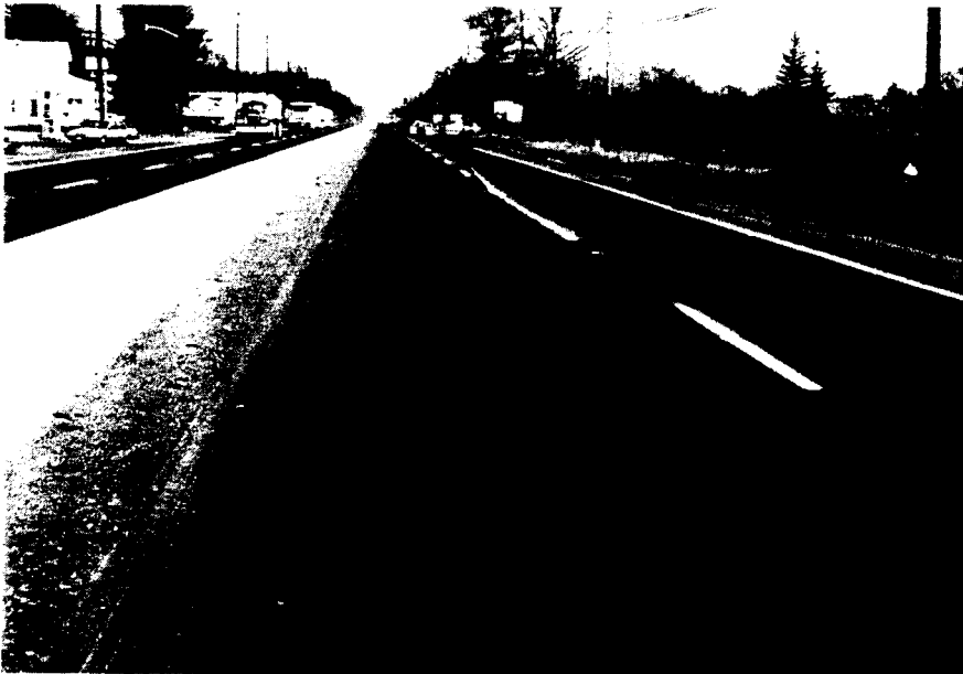
PHOTO 16 APPEARANCE OF ROUTE 1 PROJECT AFTER 10 YEARS SERVICE
