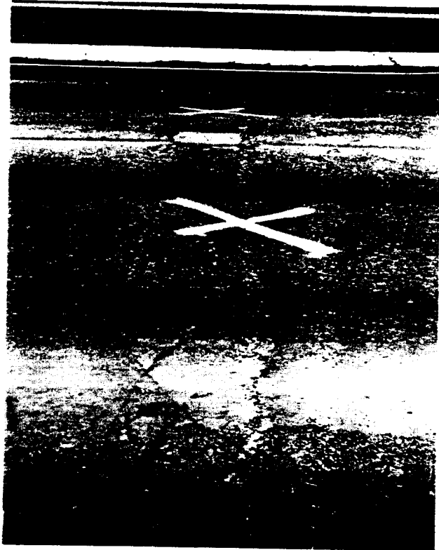
PHOTO 64 ROUTE 10 PROJECT: APPEARANCE OF OVERLAY SURFACE
