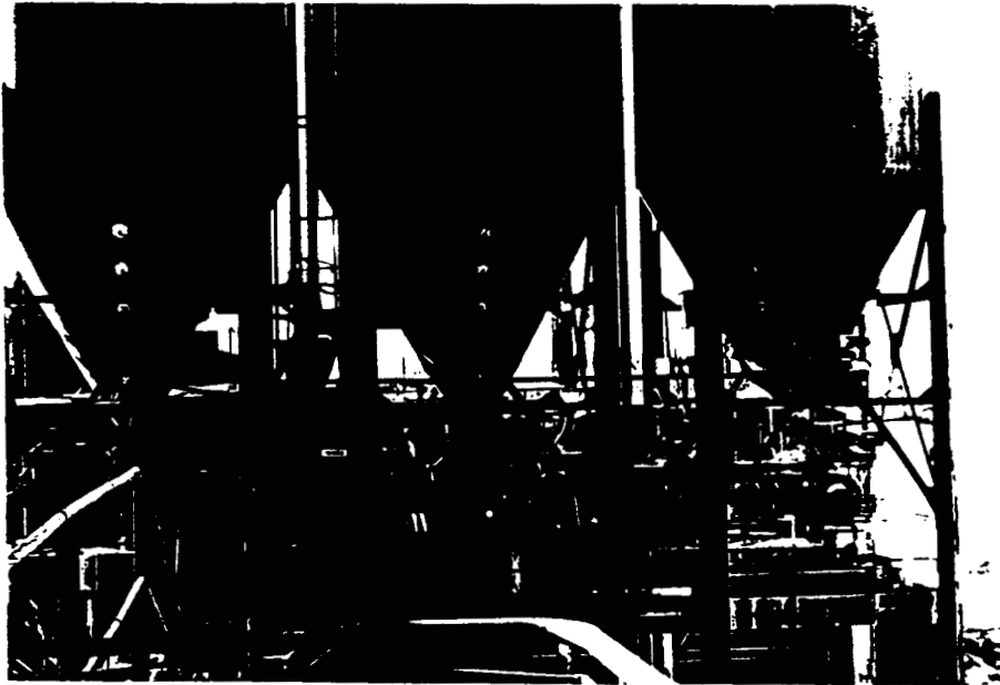
FIGURE 5. Storage Silos for Fly Ash and Lime
