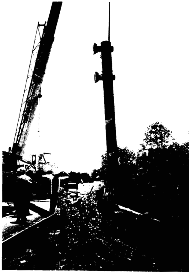
Figure 3-1 VMS Column Erection on Interstate 80.
