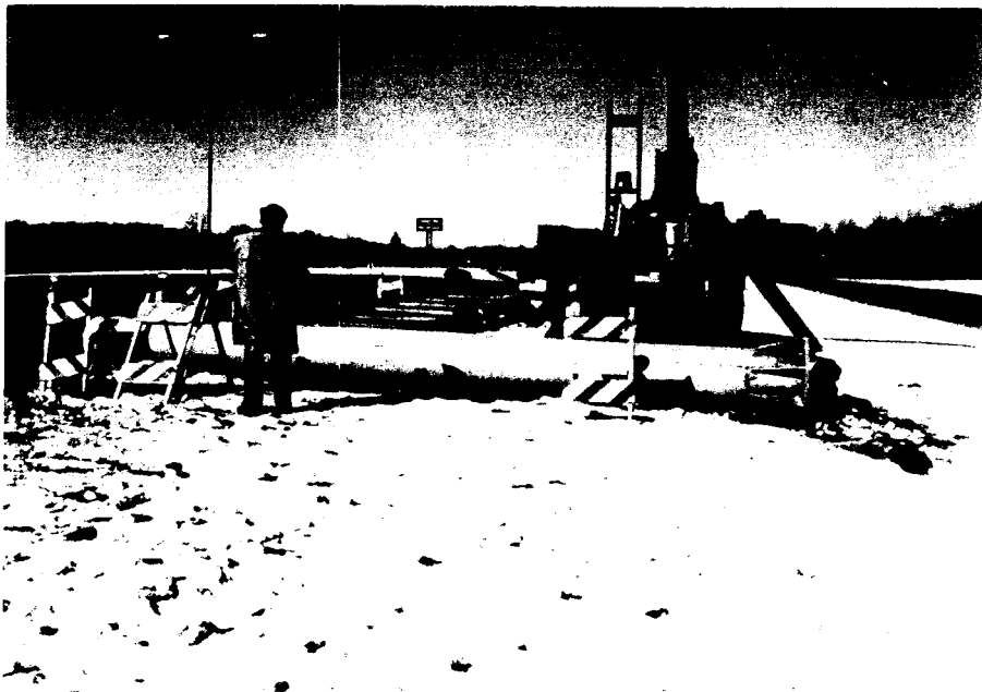
Figure 2-2 Failed VMS Support Structure Due to Anchor Bolt Fatigue
