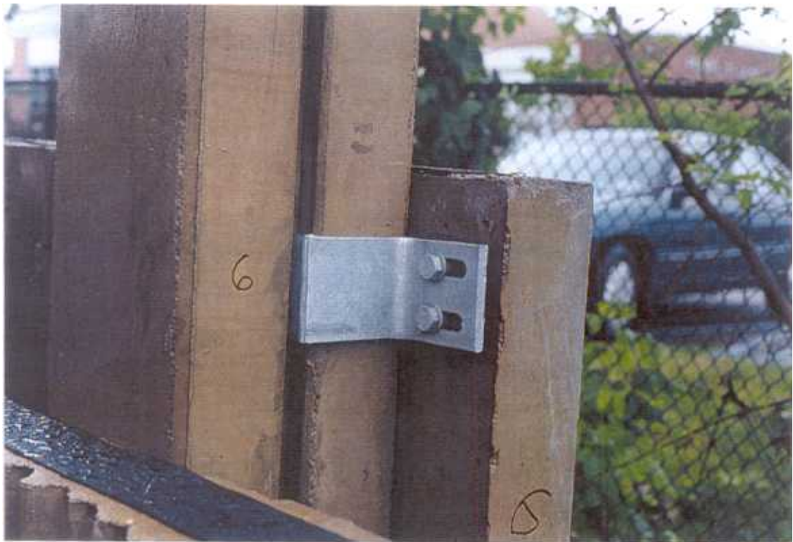
Fig. 39 Detail of angle and bolt attachment
