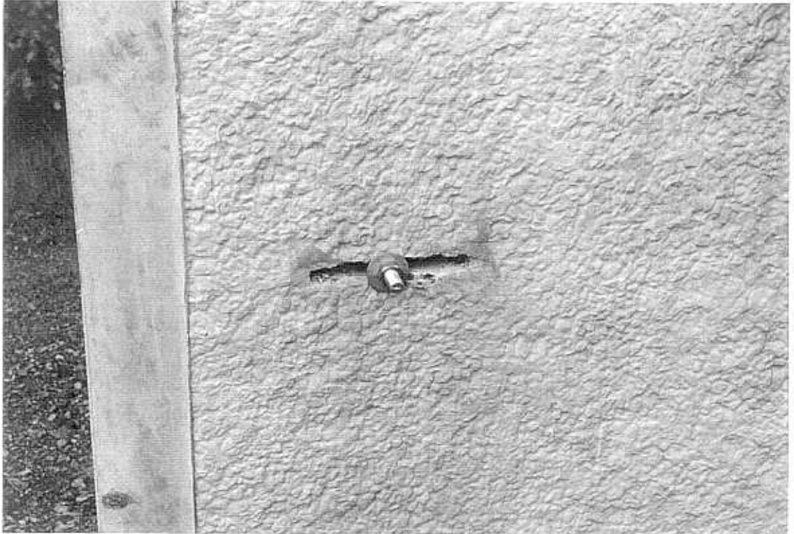
Fig. 10 Detail of T bolt in Fig. 9. Note slot mark at end of bolt to show T is set in channel.
