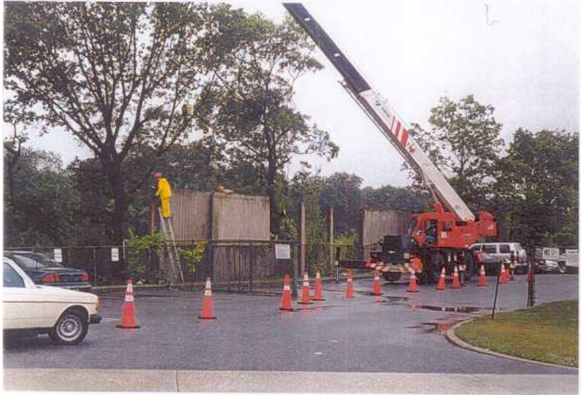
Fig. 36 NSP noise wall panel erection.
