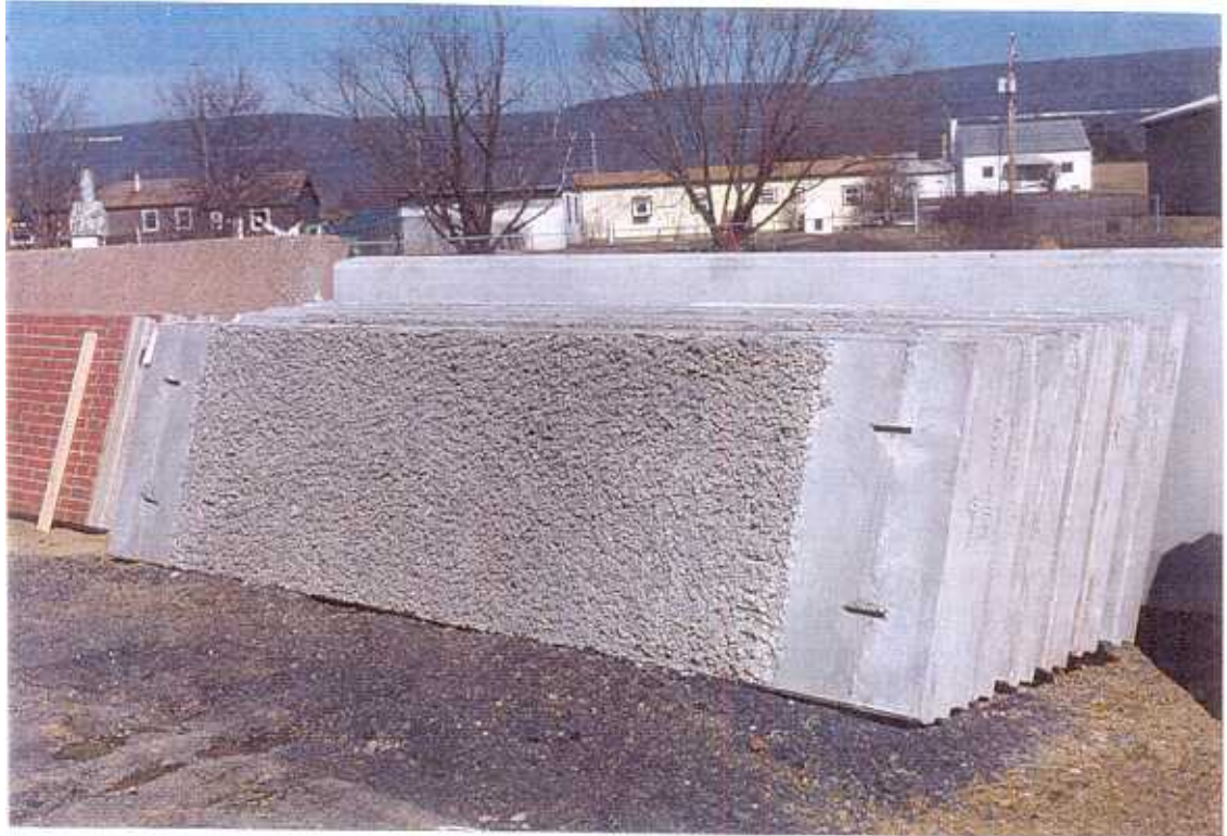
Fig. 5. Fuzzy rake finish (residential side) of 4 ft. panel with smooth end treatments which rest against the posts.
