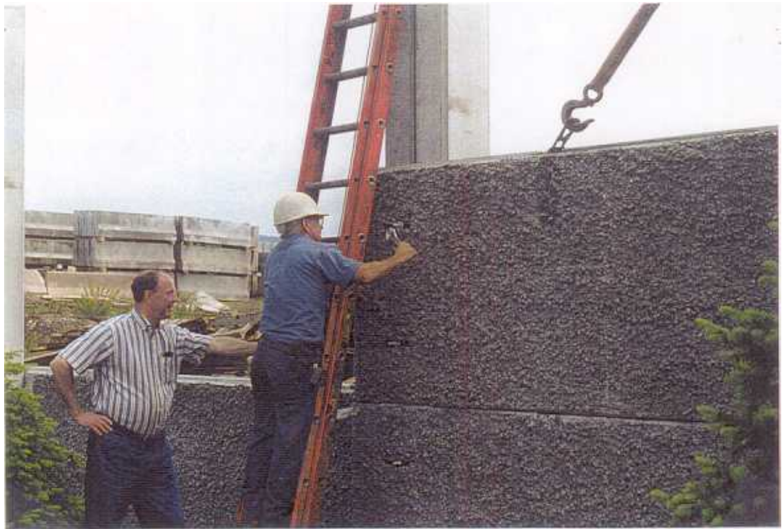
Fig. 11 Residential side bolting of panel.
