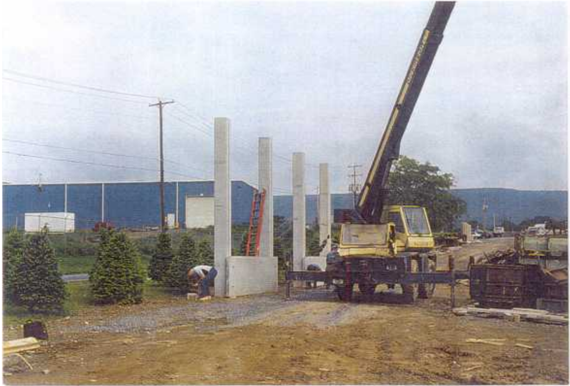
Fig. 7 Prototype posts 4@15 ft. center at CSS yard.
