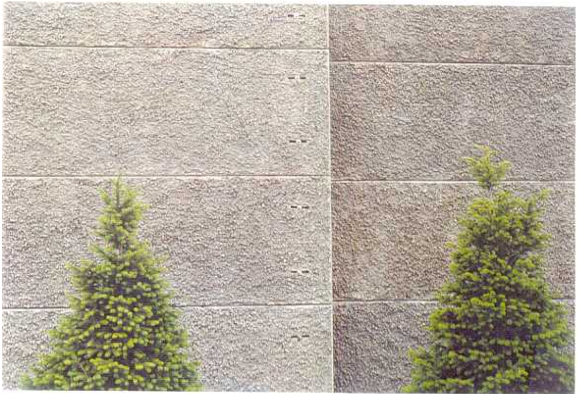
Fig. 27 Detail of T bolts on residential side.
