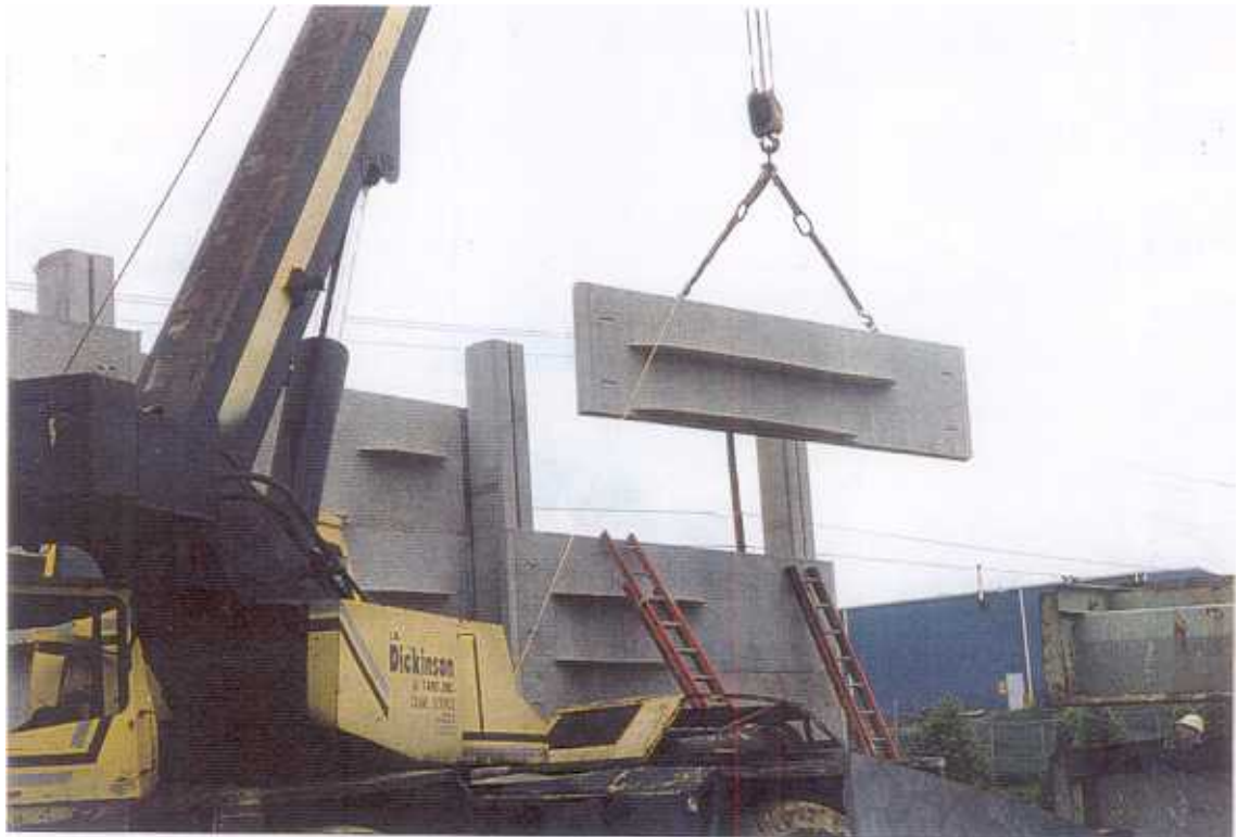
Fig. 22 Fig. 20 panel being lifted into position.
