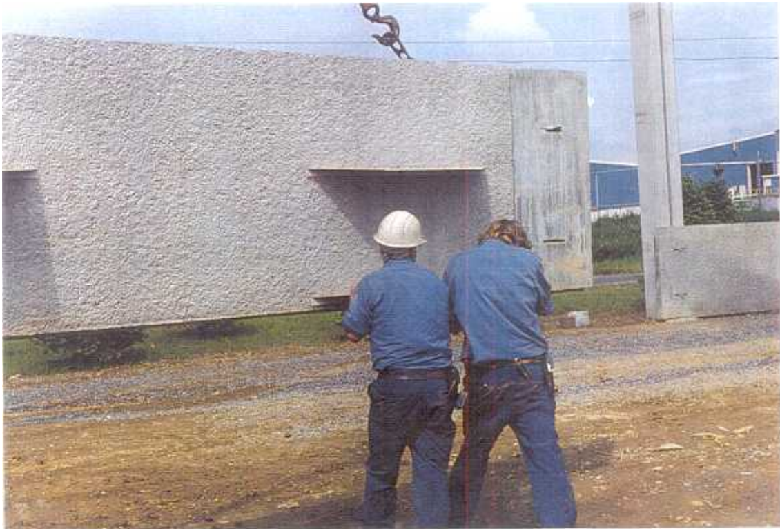
Fig. 14 Fin attachment to panels.
