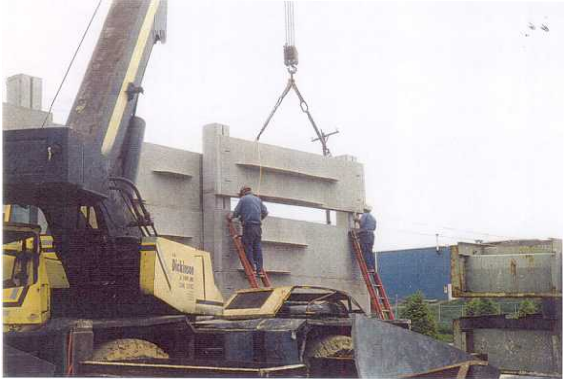
Fig. 23 Fig. 20 panel being lowered to posts.
