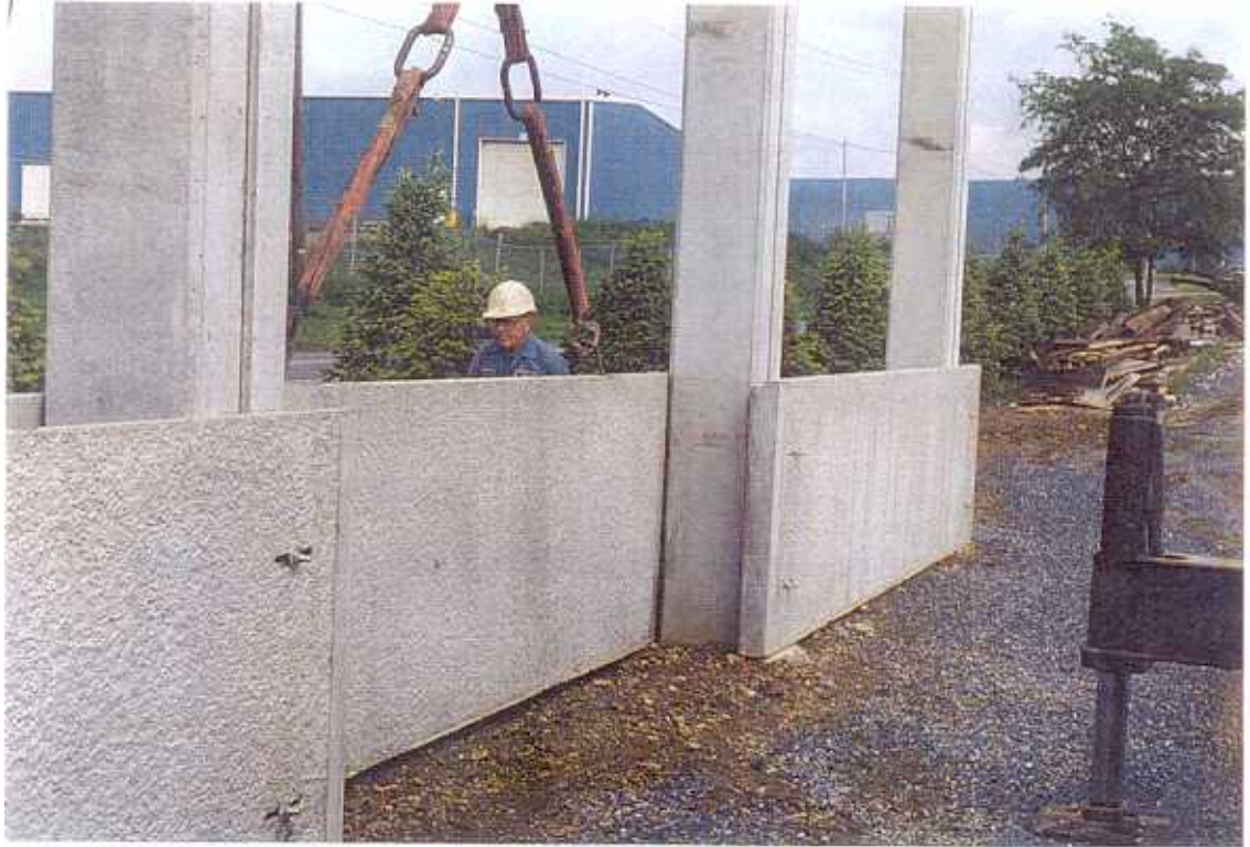
Fig. 9 Three 4 ft. bottom panels are in place.
