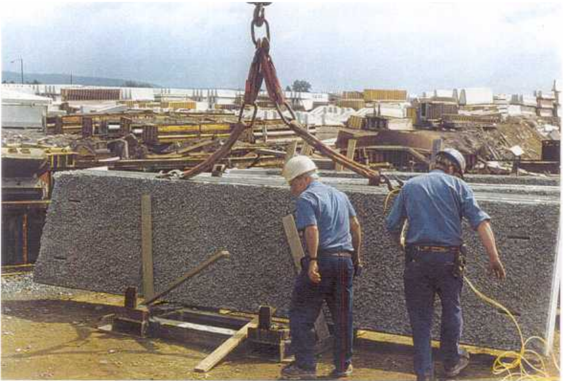
Fig. 8 Panels stacked on rack ready for erection.
