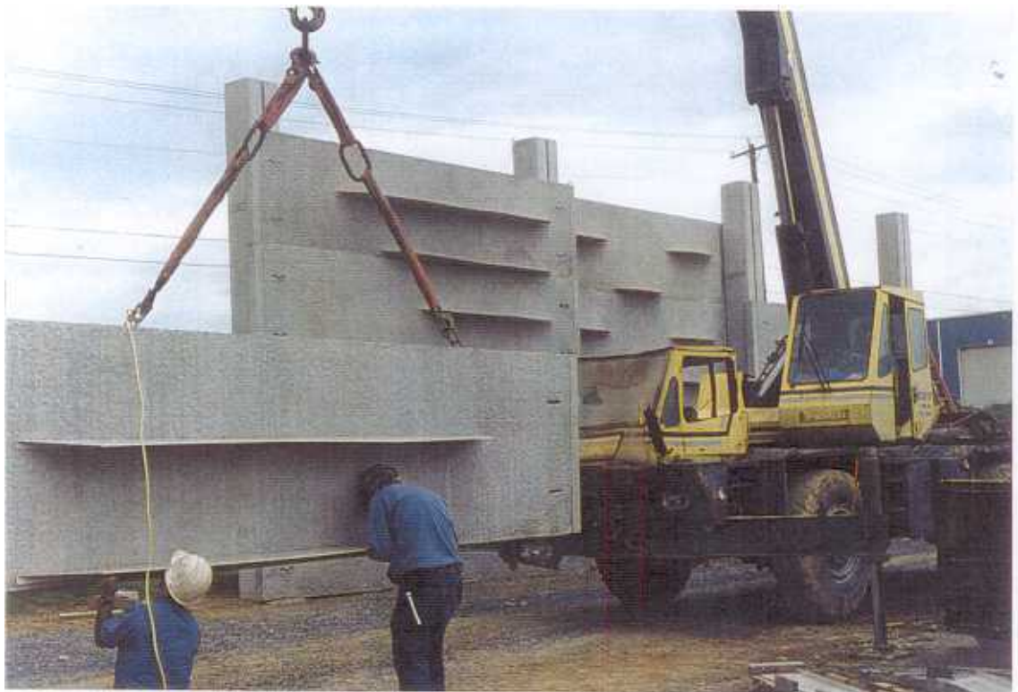
Fig. 20 8 ft. and 10 ft. fins being attached.
