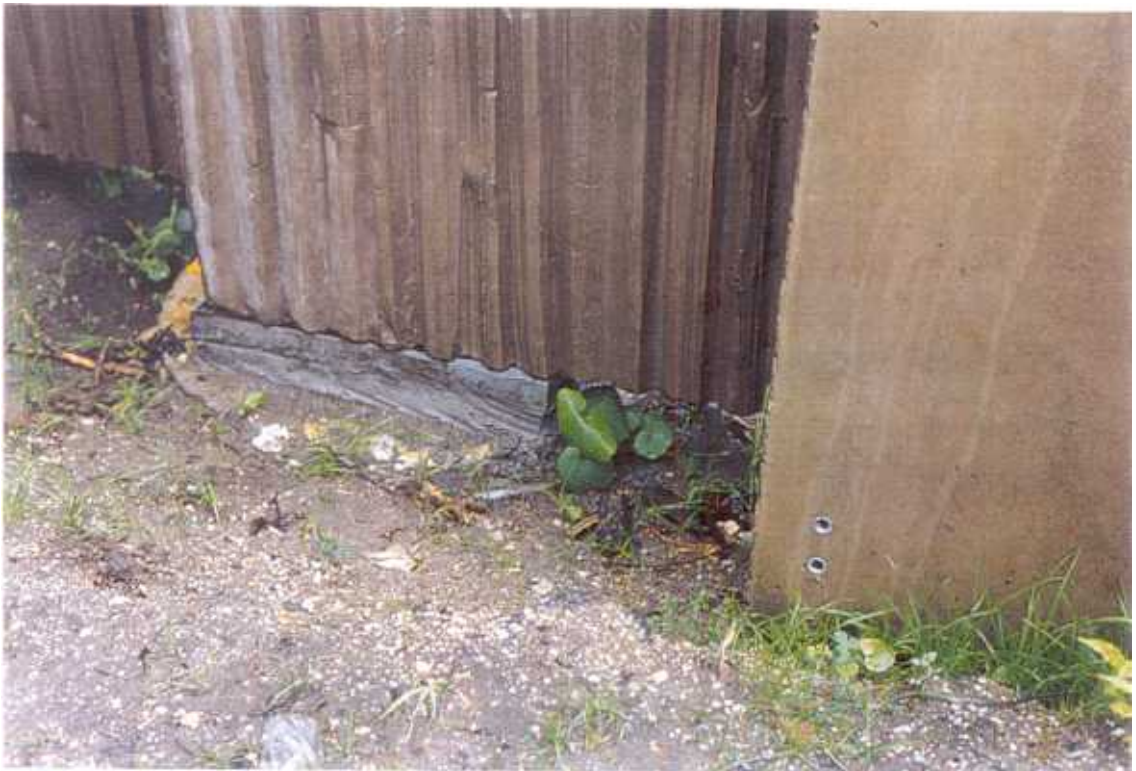
Fig. 43 Panel bolt holes at lower right.
