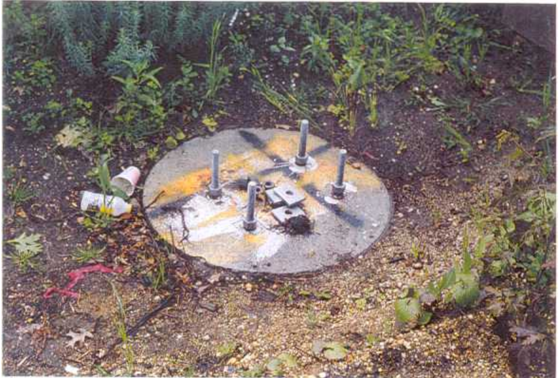
Fig. 44 Anchor bolts for post base plate.
