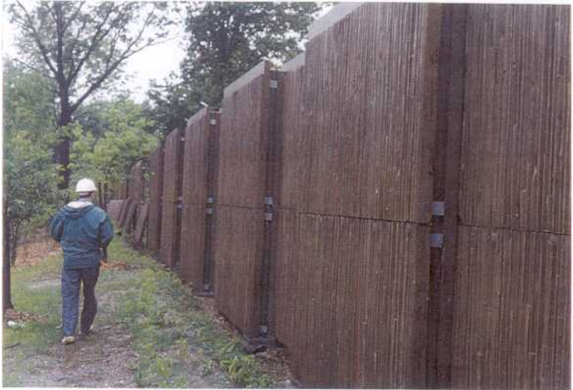
Fig. of highway side wall
