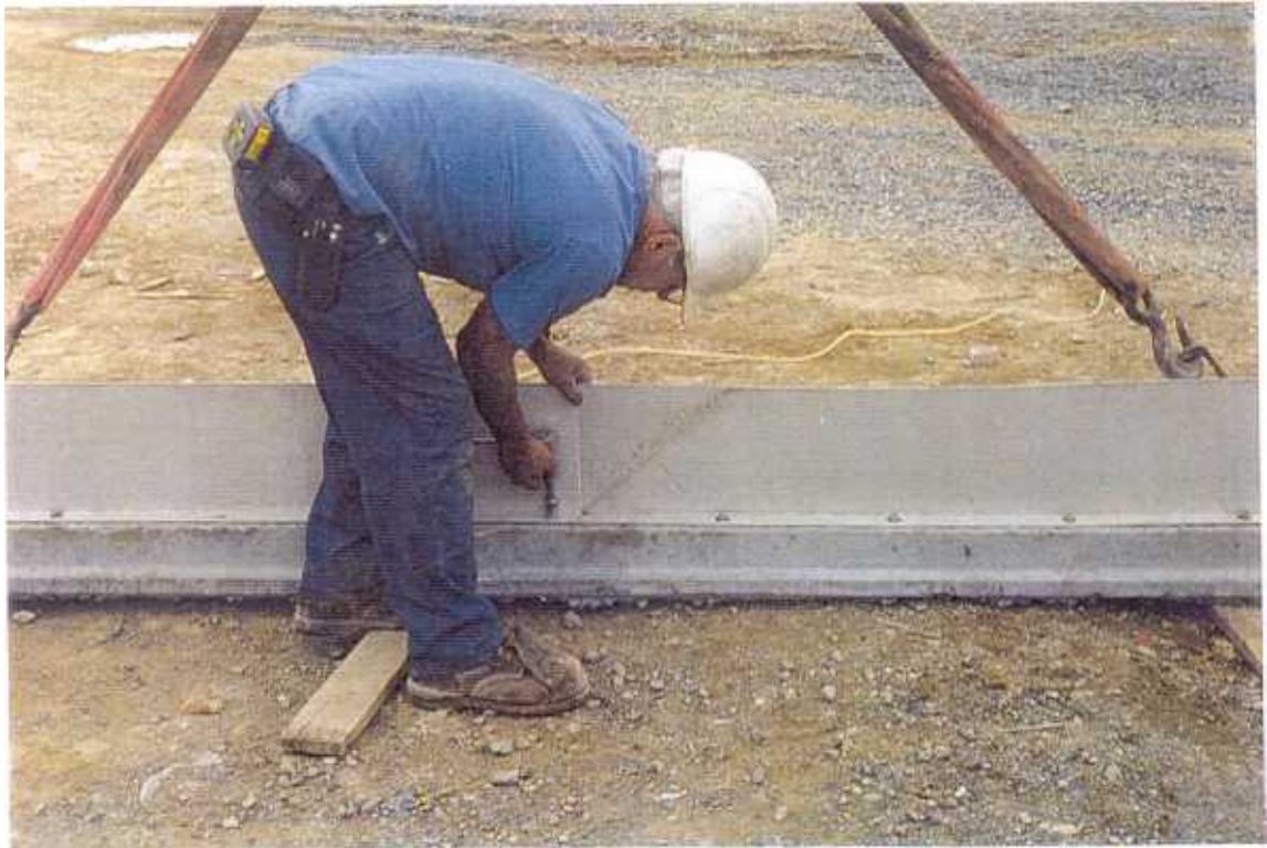
Fig. 25 12 ft. fin (6 ft. x 2) being attached.
