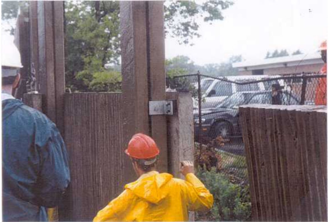
Fig. 42 Note shims used between angle and panel.
