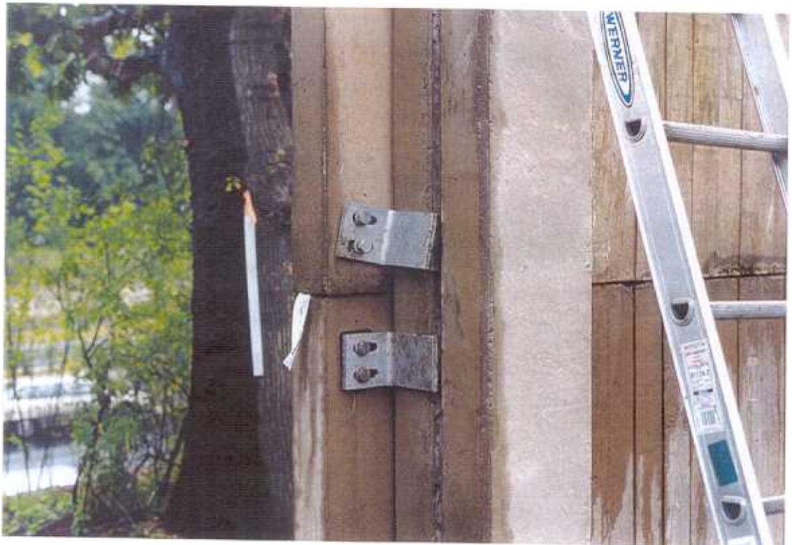
Fig. 41 Angle bracket bottom and top of post
