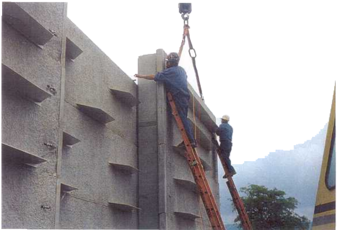
Fig. 26 Fig. 25 - 2 ft. panel being bolted to post
