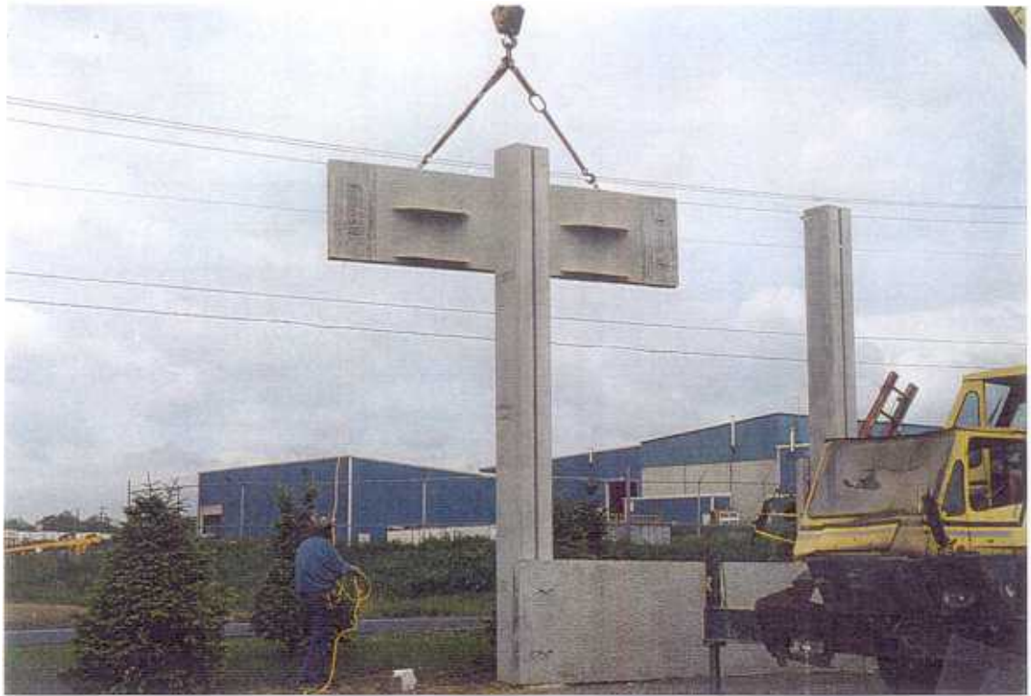
Fig. 15 Four ft. panel with four 2 ft. fins.
