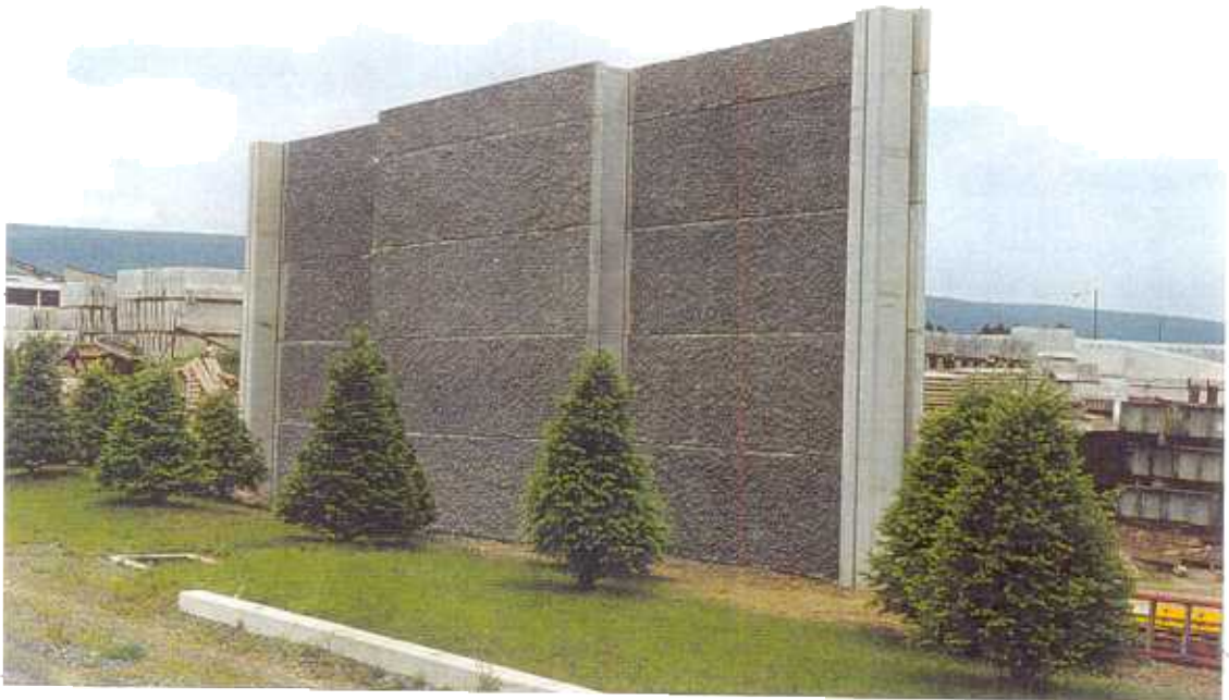
Fig. 28 Residential side completed.
