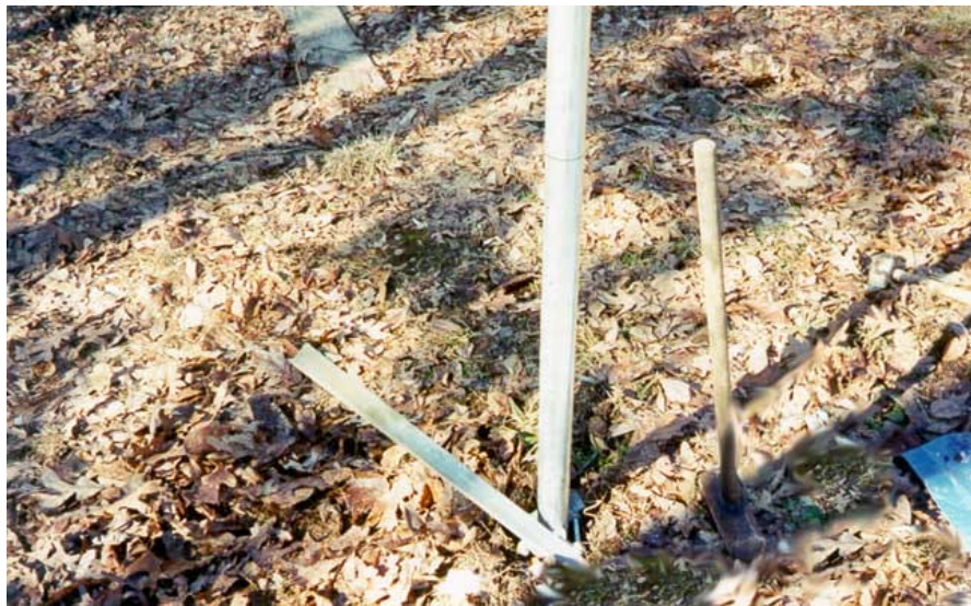
Figure 10 Photograph of driven 2.5 inch line post with one of the anchor blades driven via a sledgehammer into position.
