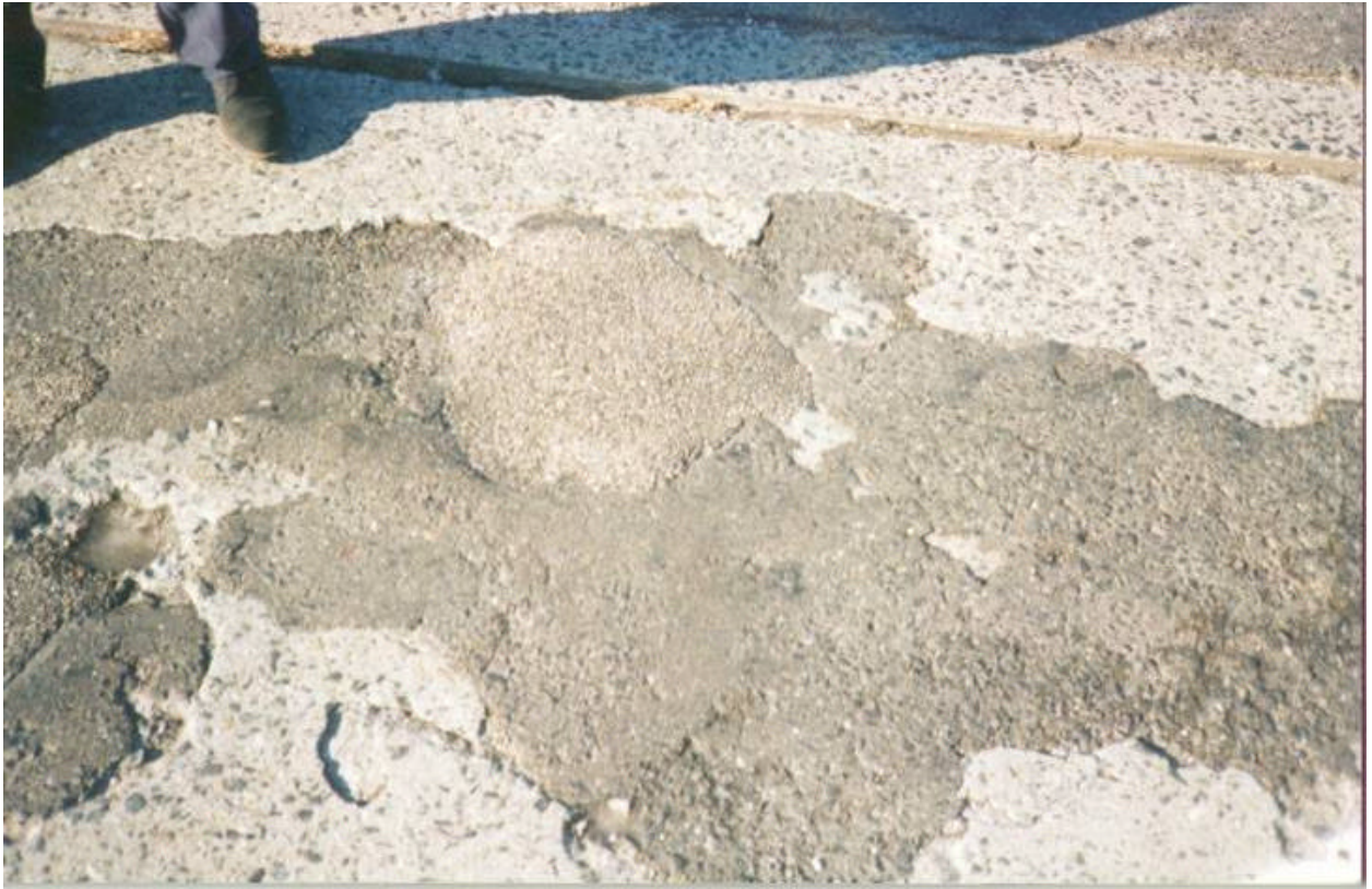
Figure 38. Performix- 2 Month Inspection, Rt. 21 SB MP 11.8 Passaic
