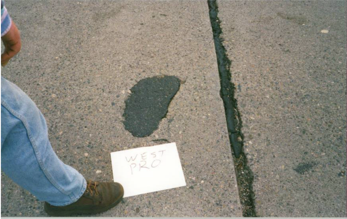
Figure 67. Wespro 6 Month Inspection, Rt. 21 SB MP 12.36 Passaic
