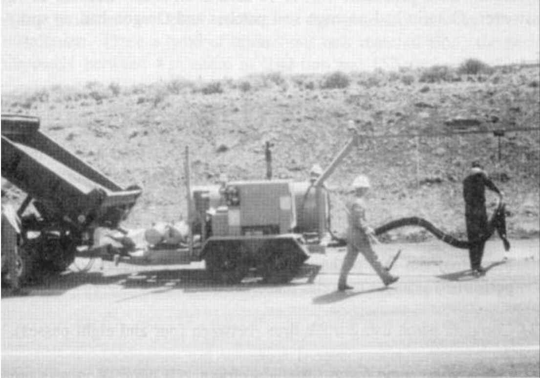
Figure 11. Spray Injection Method of Pothole Repair (5)
