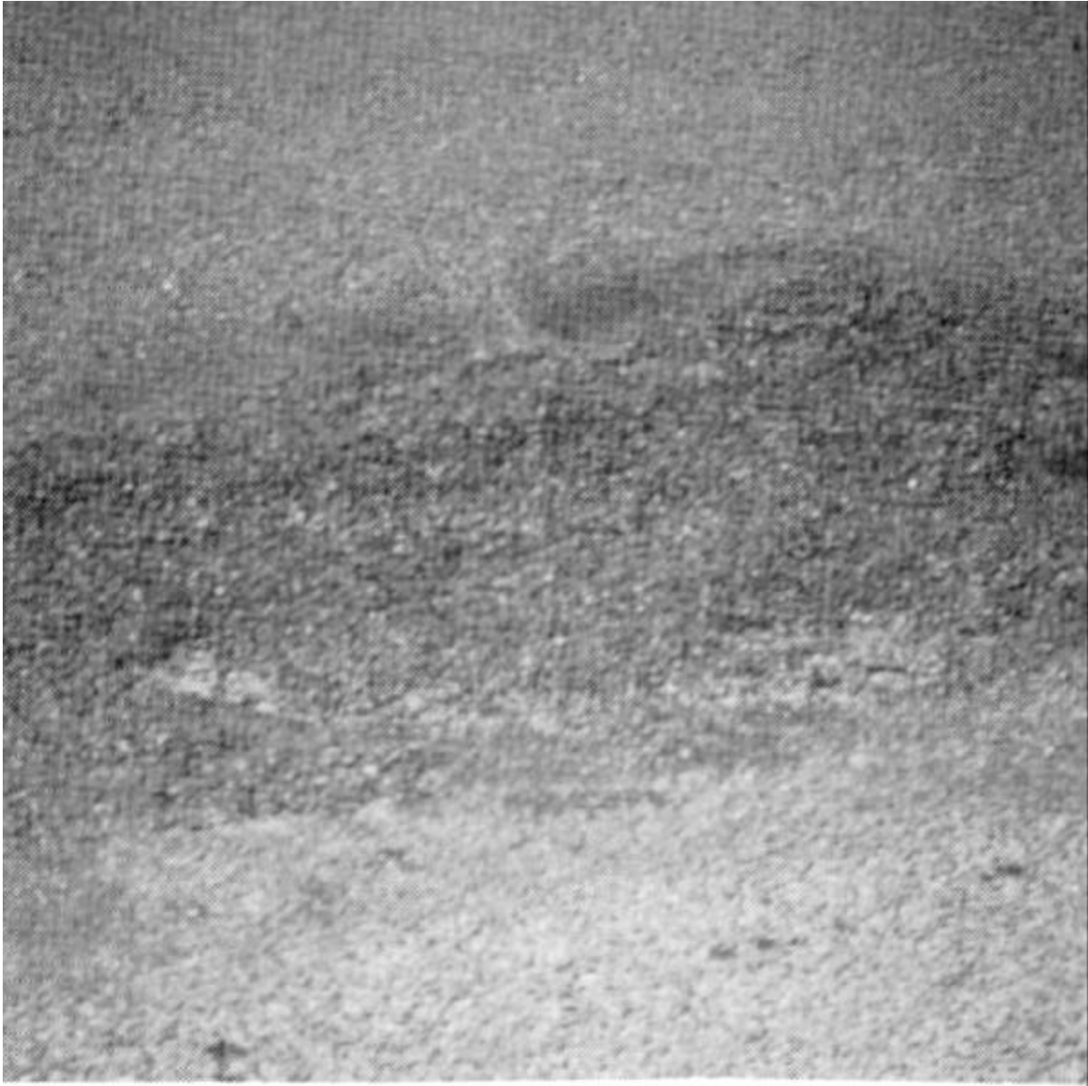
Figure 4. Raveling Distress (3)
