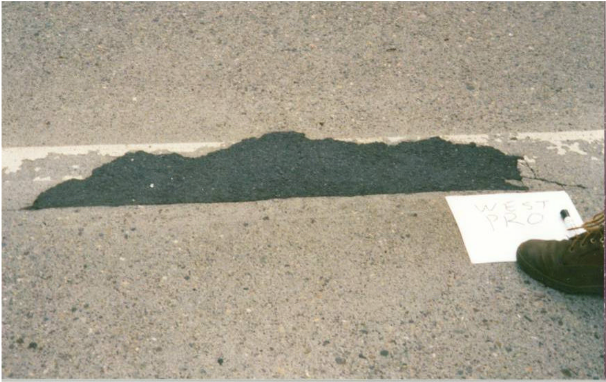
Figure 65. Wespro 6 Month Inspection, Rt. 21 SB MP 12.36 Passaic
