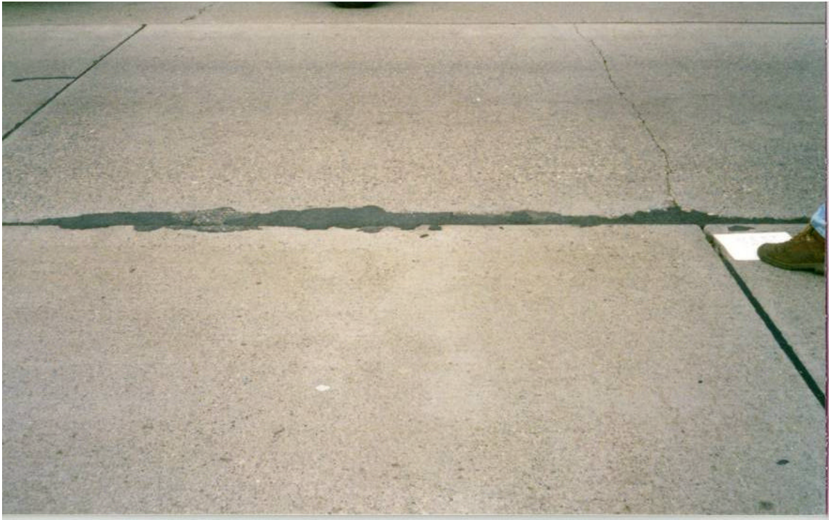
Figure 64. Wespro 6 Month Inspection, Rt. 21 SB MP 12.36 Passaic
