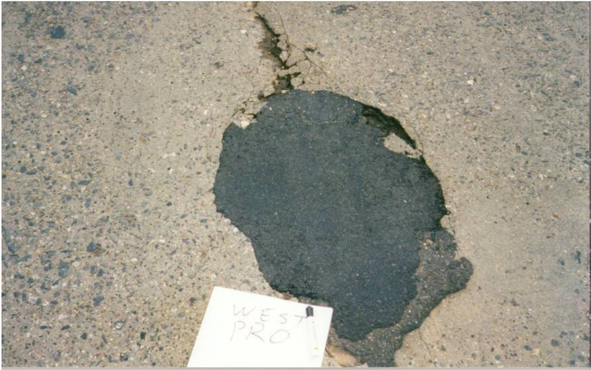
Figure 66. Wespro 6 Month Inspection, Rt. 21 SB MP 12.36 Passaic
