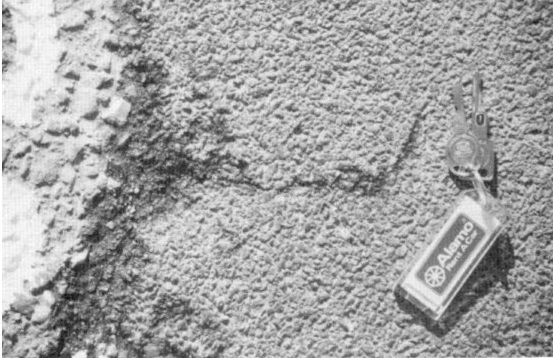
Figure 2. Cracking Distress (3)
