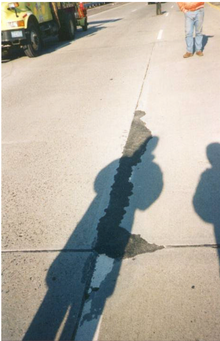
Figure 61. Wespro 2 Month Inspection, Rt. 21 SB MP 12.36 Passaic
