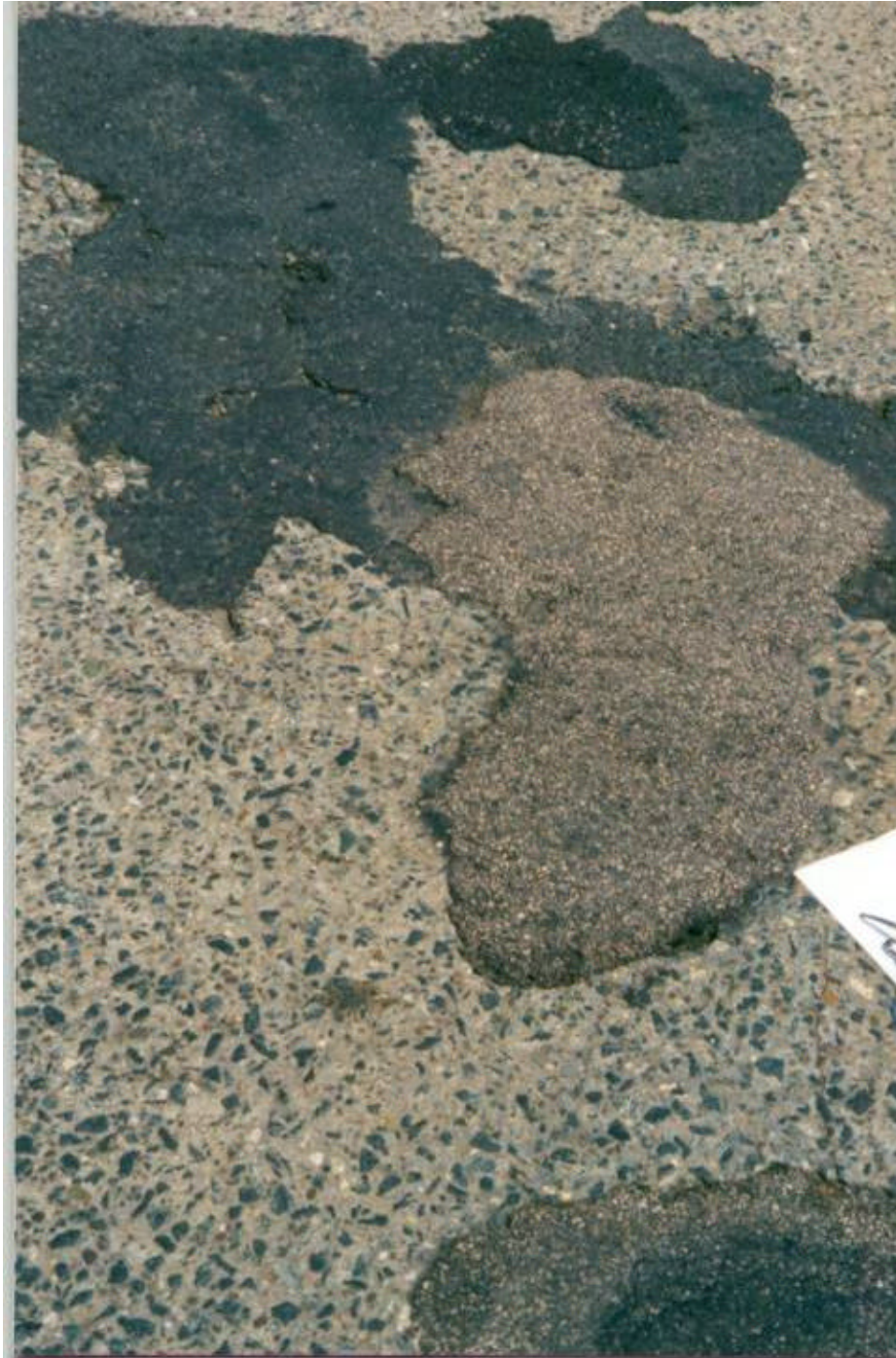
Figure 55. UPM 6 Month Inspection, Rt. 120 SB MP 2.65 over Rt. 17 East Rutherford
