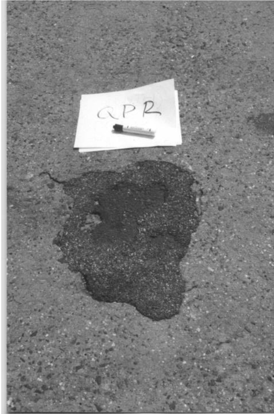
Figure 46. QPR 6 Month Inspection, Rt. 21 SB MP 12.0 Passaic
