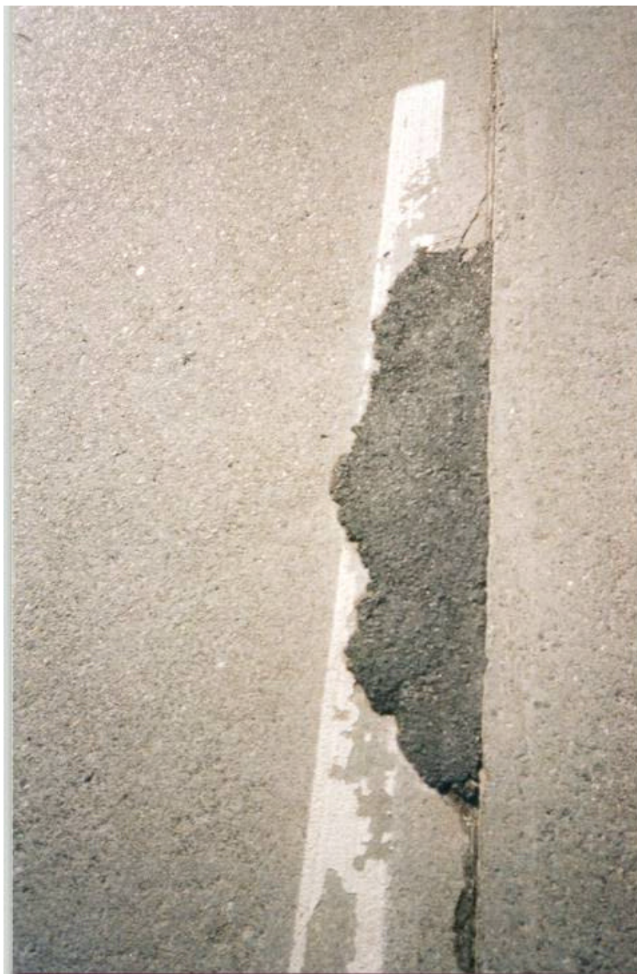
Figure 62. Wespro 2 Month Inspection, Rt. 21 SB MP 12.36 Passaic
