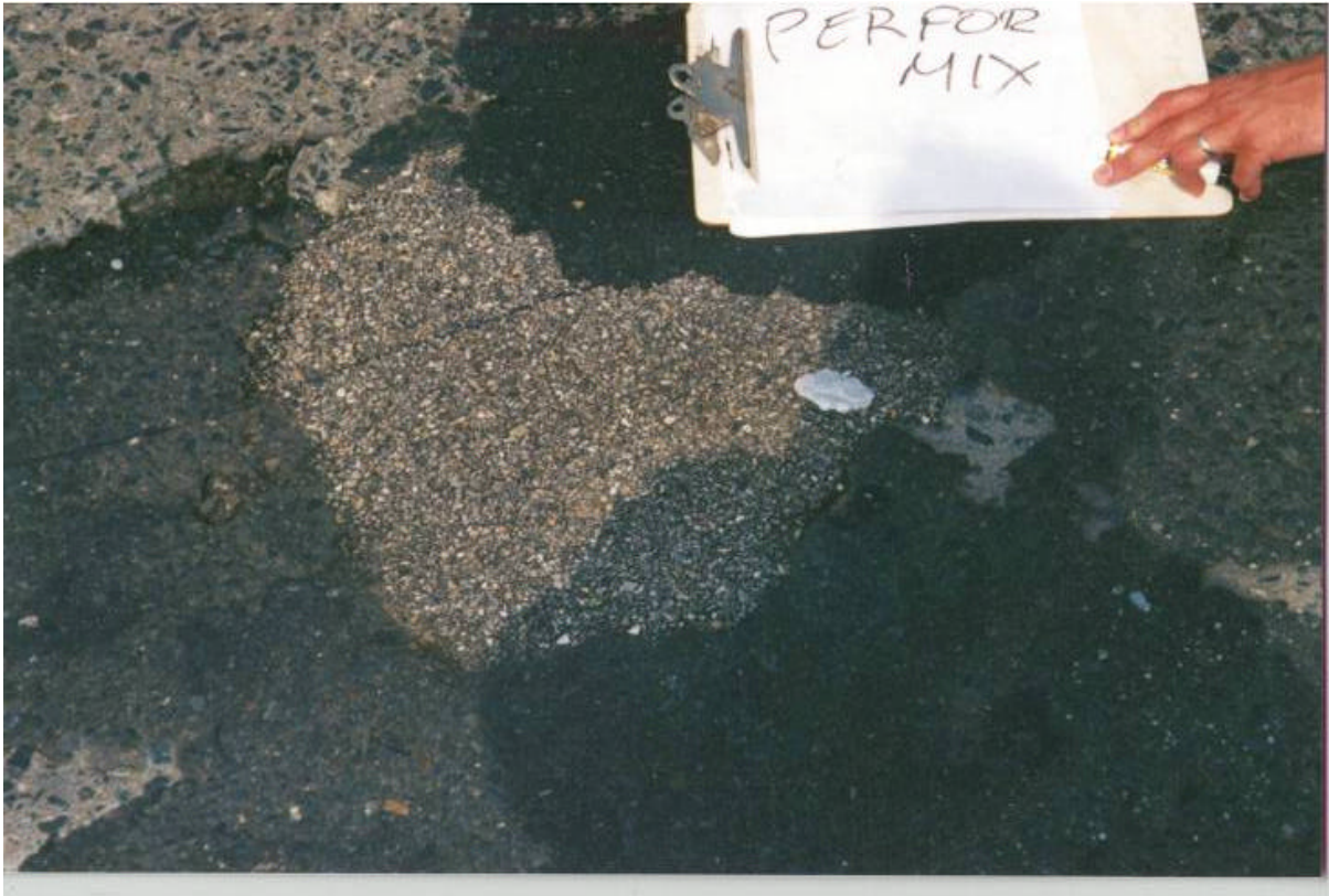
Figure 39. Performix 6 Month Inspection, Rt. 21 SB MP 11.8 Passaic
