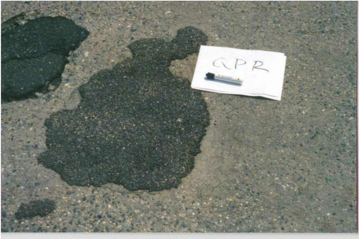
Figure 47. QPR 6 Month Inspection, Rt. 21 SB MP 12.0 Passaic
