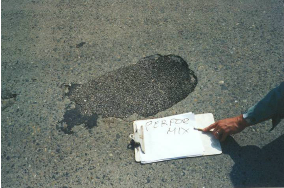
Figure 41. Performix 6 Month Inspection, Rt. 21 SB 11.8 Passaic
