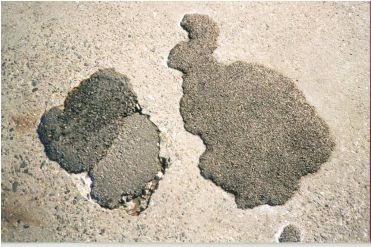
Figure 45. QPR 2 Month Inspection, Rt. 21 SB MP 12.0 Passaic
