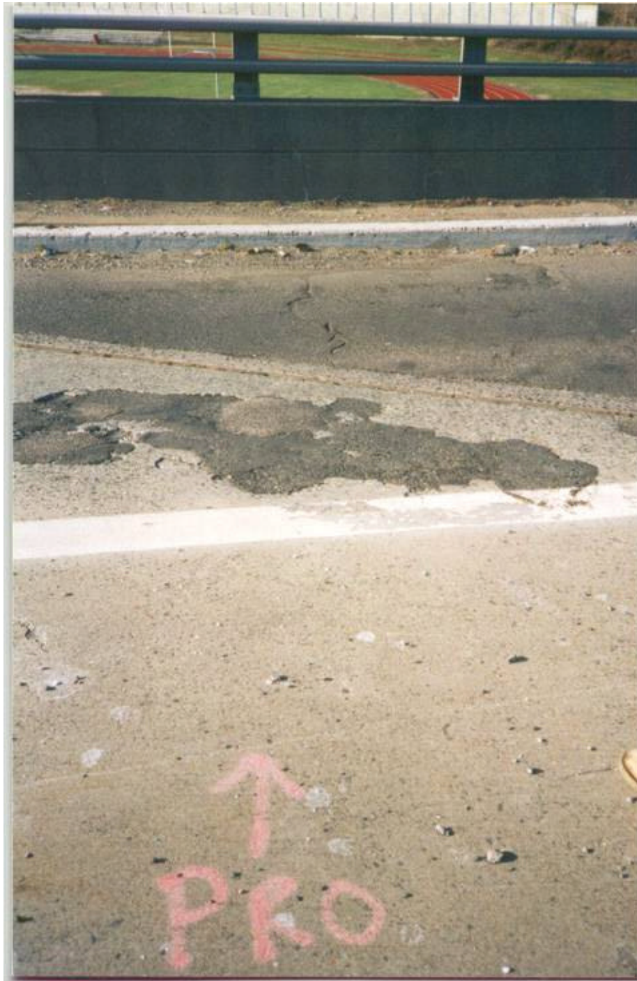
Figure 60. Wespro 2 Month Inspection, Rt. 21 SB MP 12.36 Passaic
