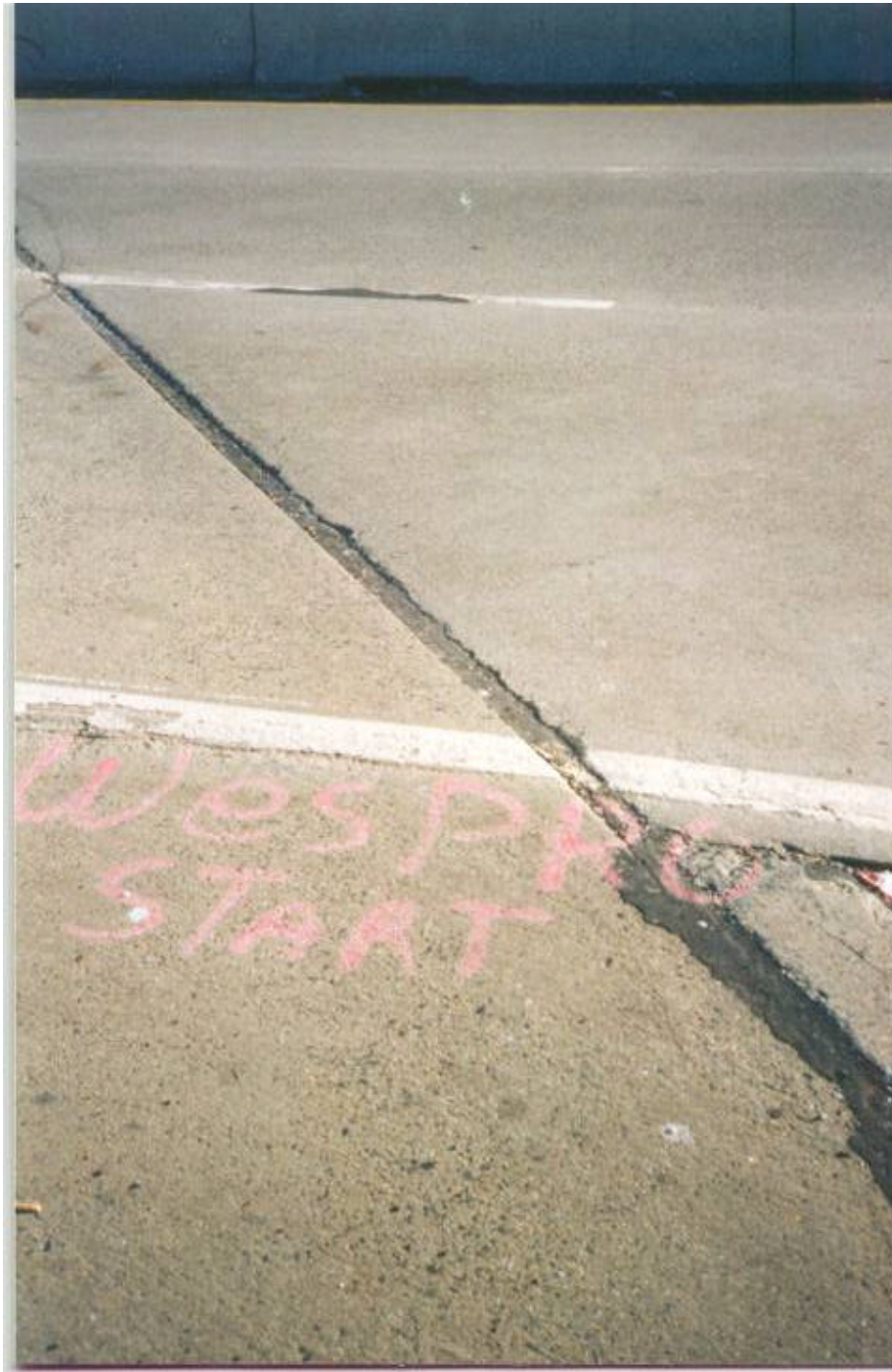
Figure 63. Wespro 2 Month Inspection, Rt. 21 SB MP 12.36 Passaic
