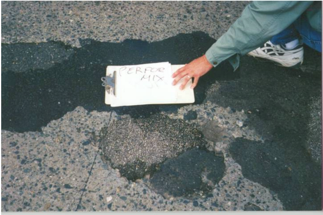
Figure 40. Performix 6 Month Inspection, Rt. 21 SB MP 11.8 Passaic
