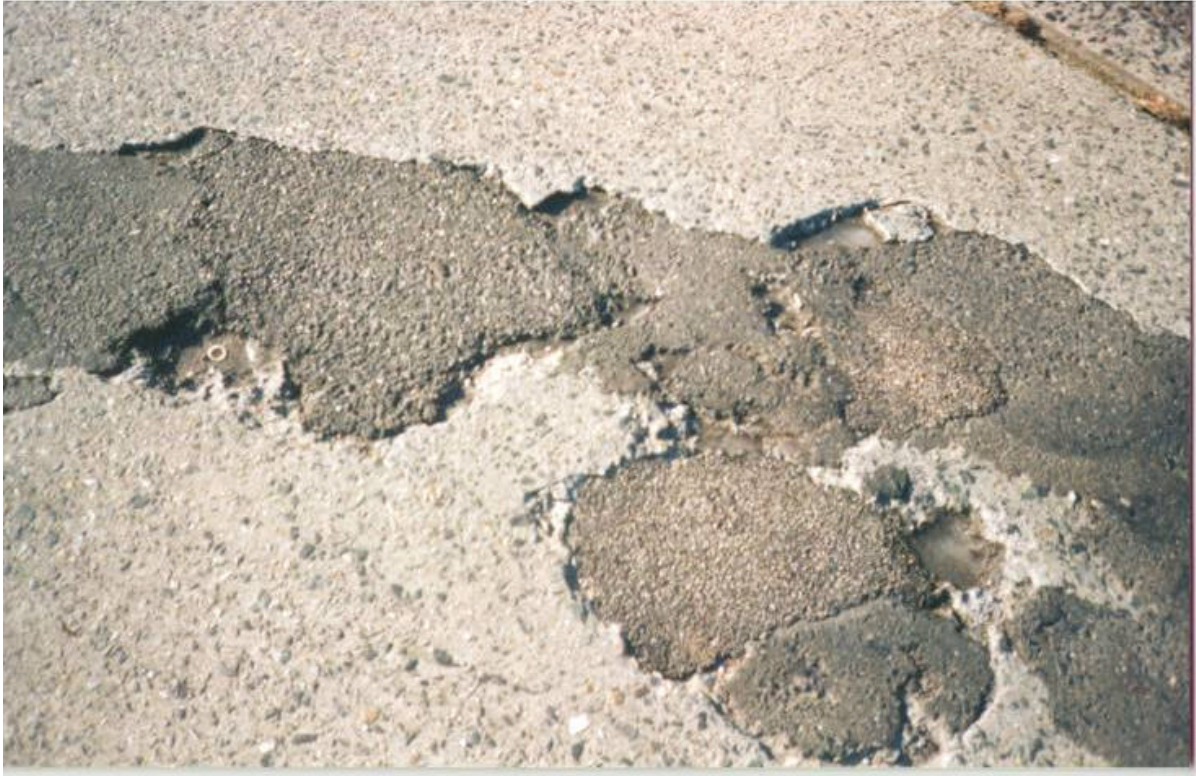
Figure 43. QPR 2 Month Inspection, Rt. 21 SB MP 12.0 Passaic
