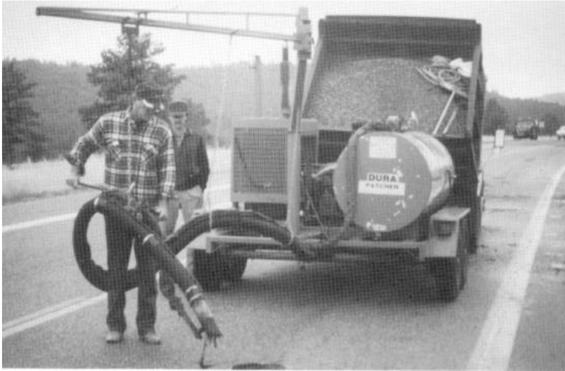
Figure 10. Spray Injection Method of Pothole Repair (5)
