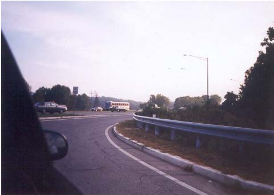
Figure 3.6 - Ramp 306 on I-80 (Route 615/Howard Boulevard)
