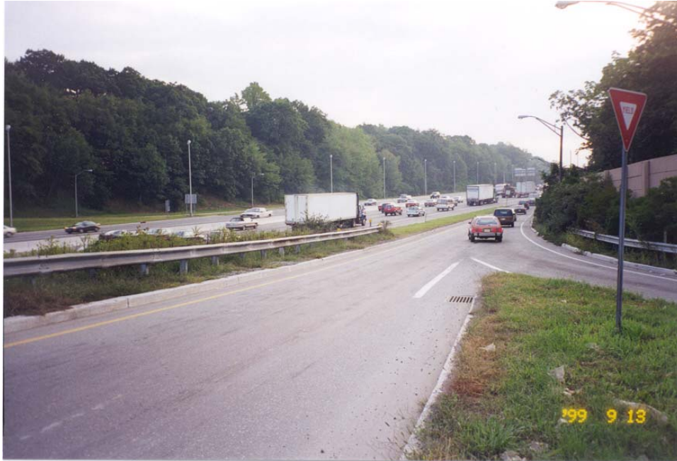
Figure 3.3 - Ramp 375 on I-80 (Route 513/Hibernia Avenue)
