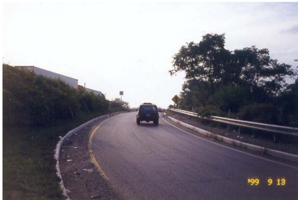
Figure 3.4 - Ramp 376 on I-80 (Route 513/Hibernia Avenue)
