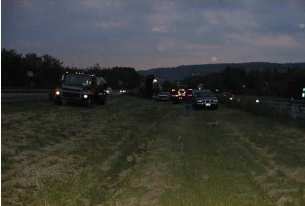
Plate 5: Typical Staging Area- Milling and Paving Project
