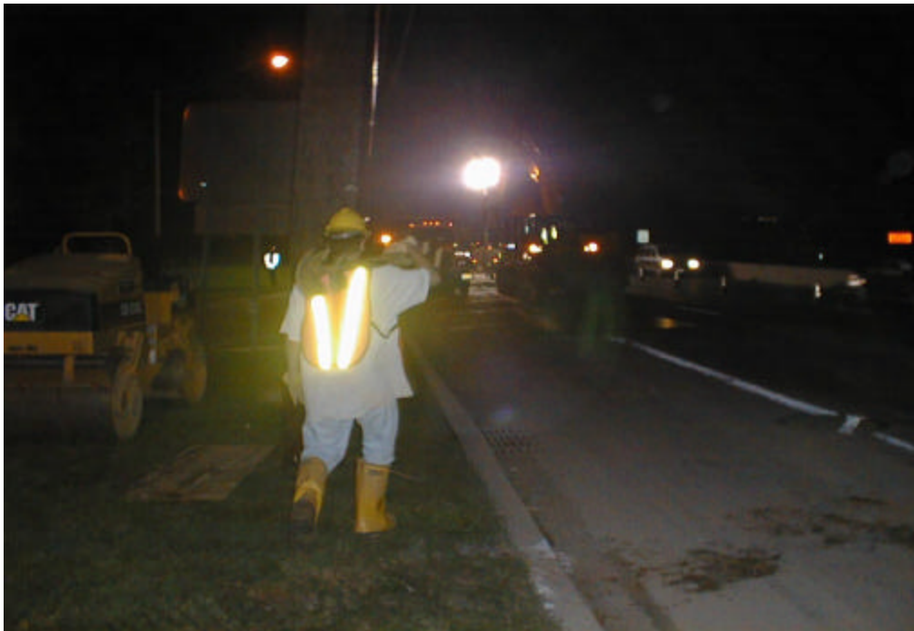
Plate 2: Typical Working Area- Fiber Optics Project
