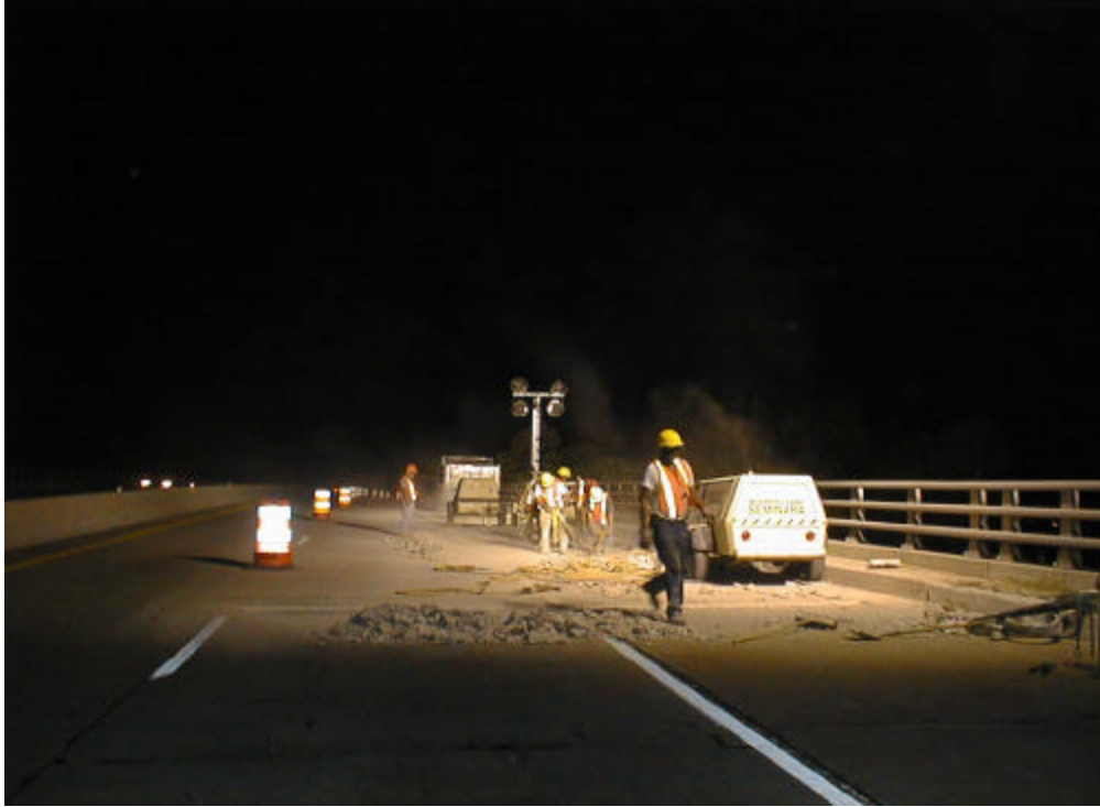
Plate 1: Typical Working Area- Bridge Rehabilitation Project
