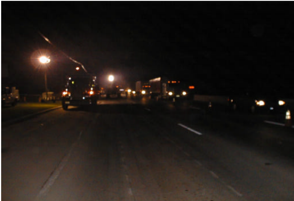
Plate 3: Lighting in Working Area- Fiber Optics Project
