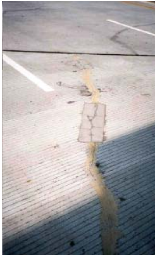
Figure 108. Repaired transverse crack (Bridge No. 1143-170).
