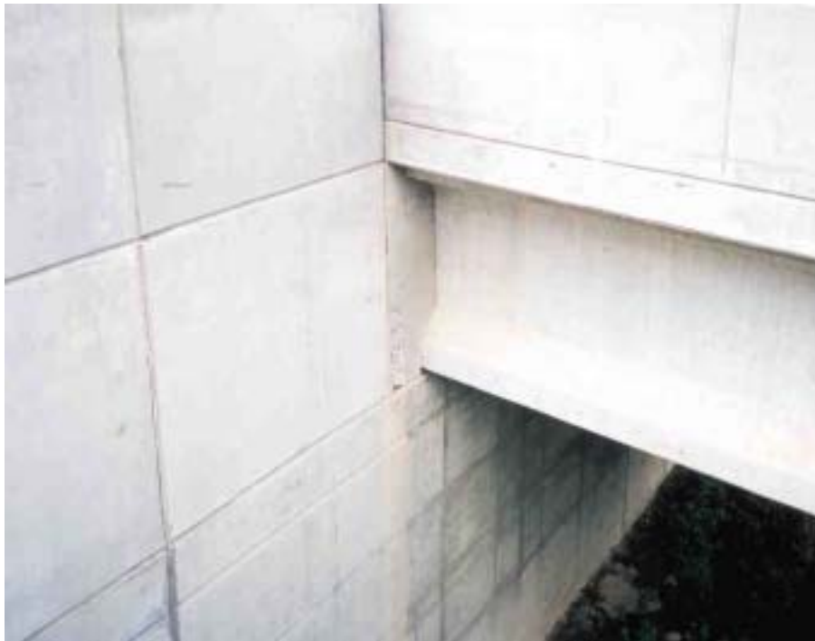
Figure 105. Girders embedded in end diaphragm (Bridge No.1143-168).
