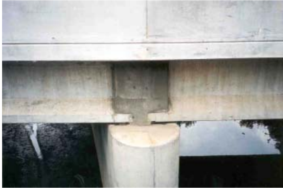
Figure 106. Continuity joint (Bridge No. 1143-168).
