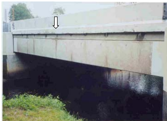
Figure 1. Corrosion due to transverse deck cracks in a bridge in New Jersey.
