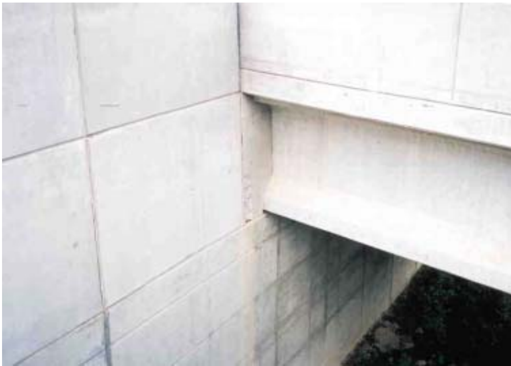
Figure 10. Boundary condition: girders are bounded.
