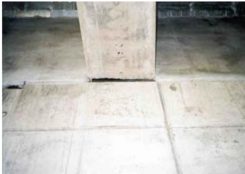
Figure 113. End diaphragm (Bridge No.1143-176).
