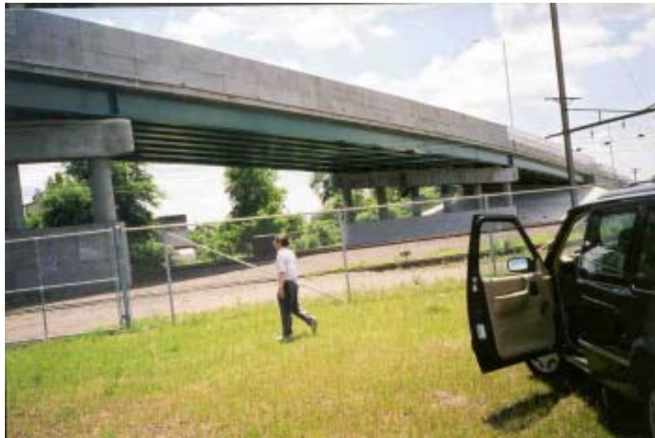
Figure 117. A view of the bridge (Bridge No.1149-168).
