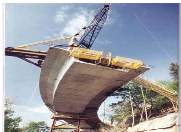
Figure B1. Segmental Bridge Construction
