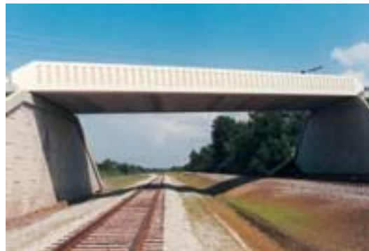
Figure B8. Through Girder Bridge (Sedley Bridge, Indiana)
