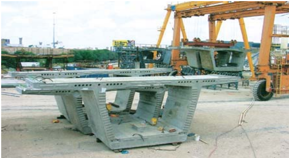
Figure B3. Segmental Components (Post-Tensioning Ducts Visible)
