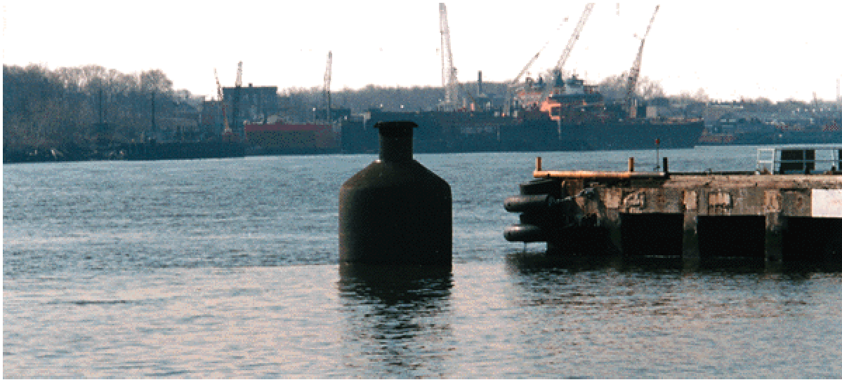
Figure A17. Floating Donut Fender at New York Port
