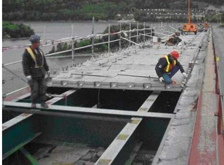
Figure B1. Full Depth Concrete Bridge Deck Panels
