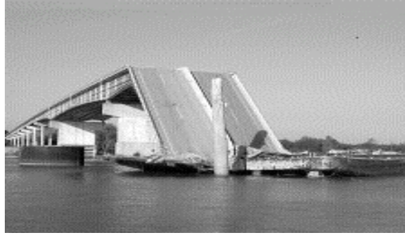
Figure A1. I-40 Bridge, Arkansas River
