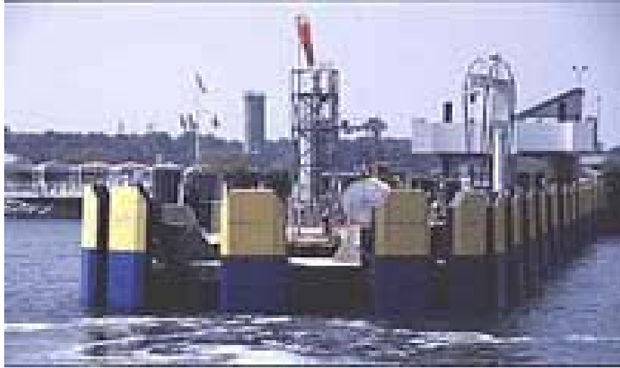
Figure A18. Pier End at Lewis, DE Ferry
