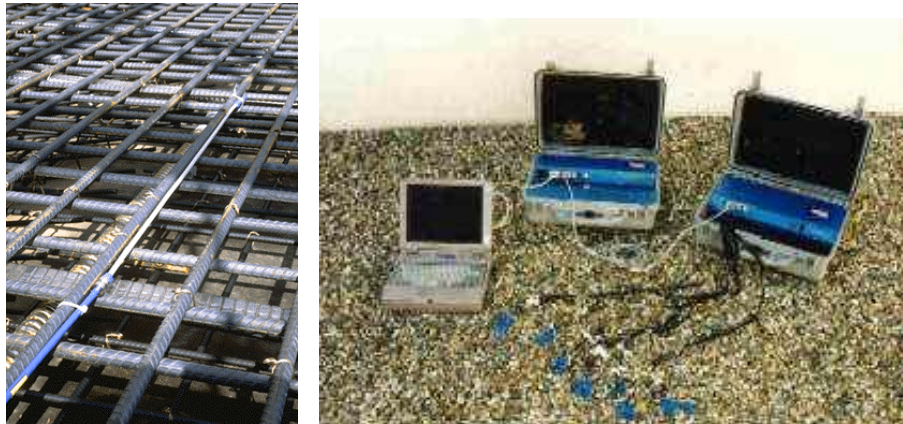
Figure C40. SOFO System Setup
