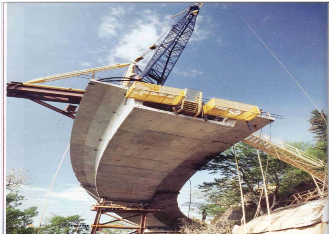
Figure B2. Construction of a Segmental Bridge
