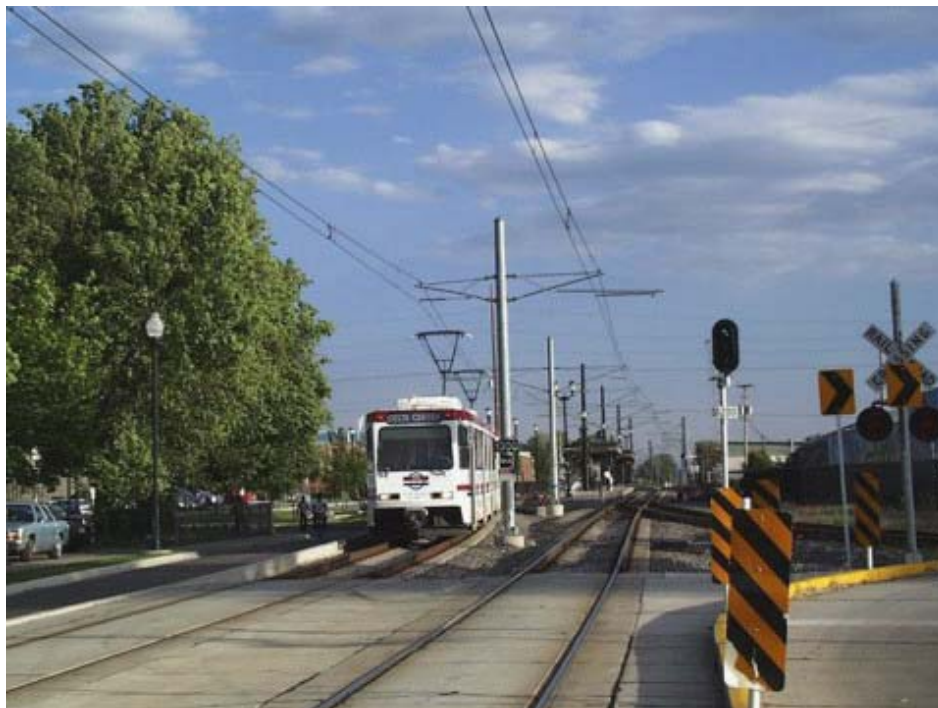
Figure 37. Freight lead connection to LRT tracks
