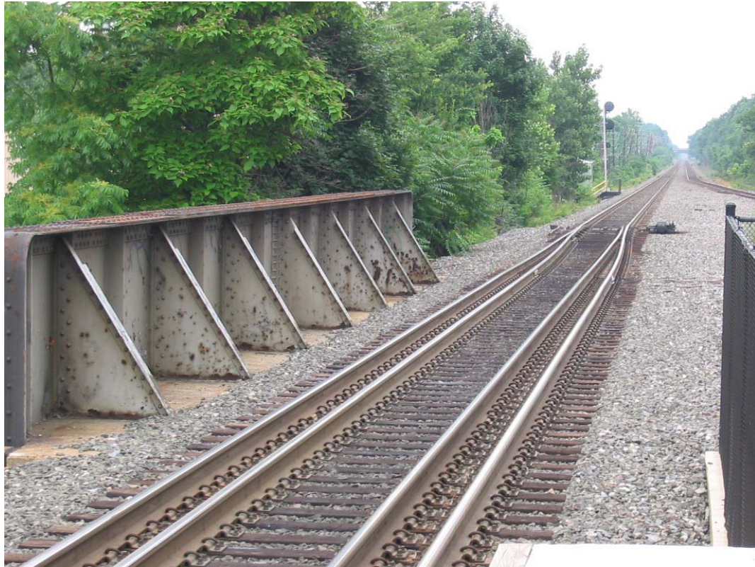
Figure 29. Gauntlet Track at Union Station, NJ
