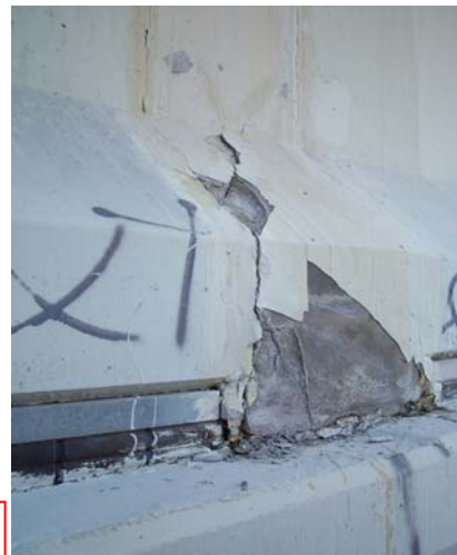
Diaphragm Cracking
