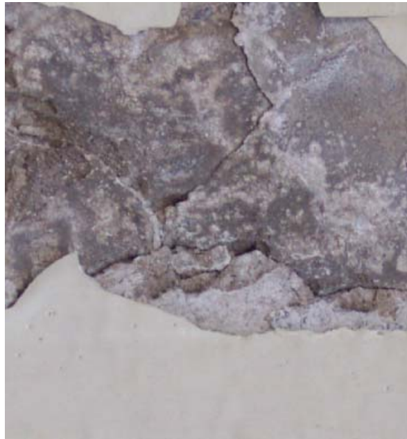
Figure 25. A close-up of the crushed concrete at fascia beam (Rt. 1&9, Newark).
