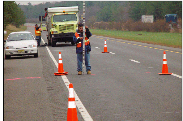
Rod and Level Survey
