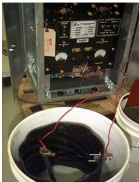
(a) Culvert1-Connected to the Rectifier
