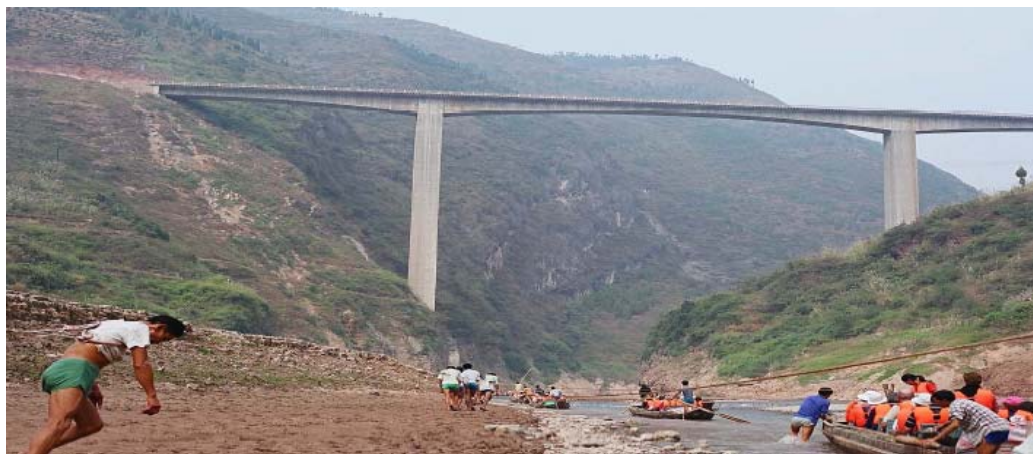
Figure 13: Vulnerability of bridge piers in remote areas.
