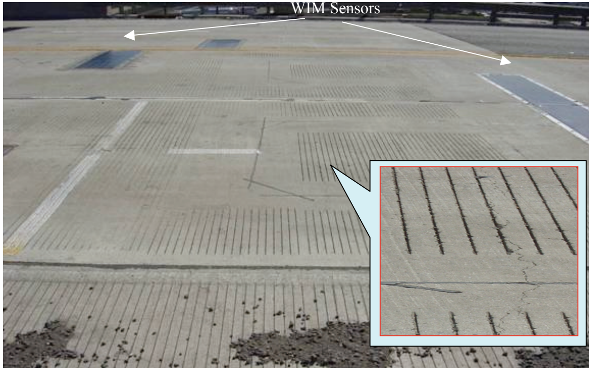
Figure 2. Crack Location and orientation in new Approach Slab at the Doremus Avenue
