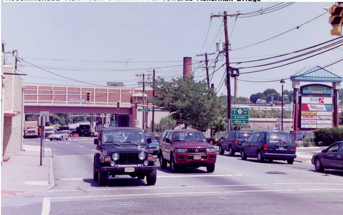
Post- Construction View from Cheever Ave. Towards Ackerman Bridge
