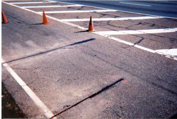
Photograph of the completed WIM installation at the Route 287 weigh station.
