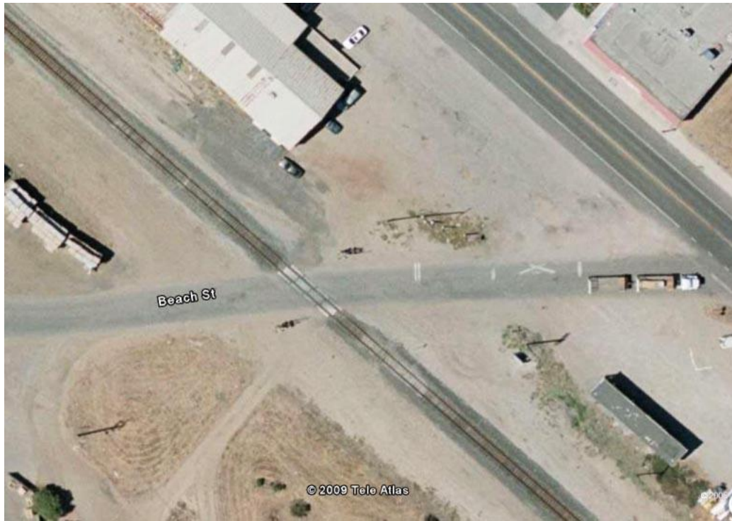
Figure 40. Railroad crossing in Oceano, CA with clear field of view
