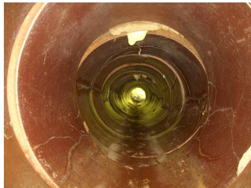
Figure 4. Clay pipe culvert: view of interior
