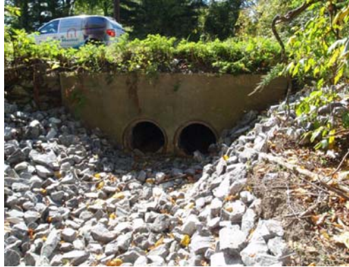
Figure 2. Clay pipe culvert: view of inlet side
