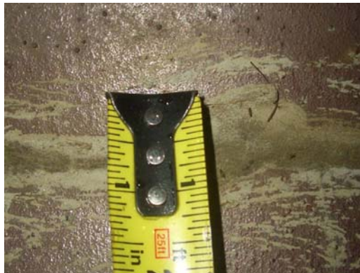
Figure 7. Repair of a winding small gap caused by pipe settlement
