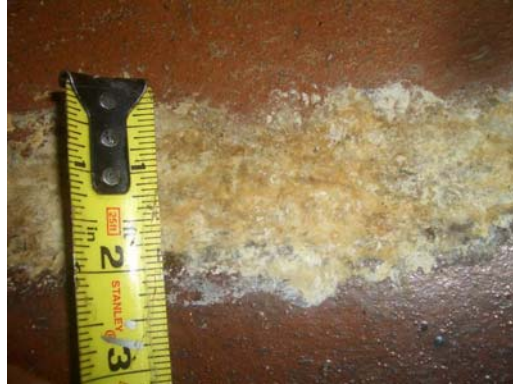
Figure 9. Repair of larger gap caused by pipe settlement
