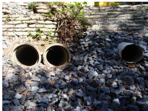
Figure 3. Clay pipe culvert: view of outlet side
