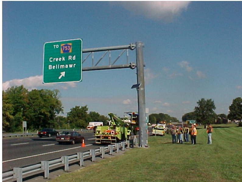
NJDOT maintenance crew deploying a traffic sensor in South Jersey
