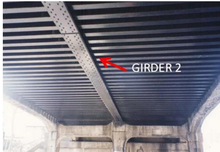
Figure 22. General view of Span 2 superstructure and underside of Girder 2 of the Main Line MP 15.95 Bridge (25)
