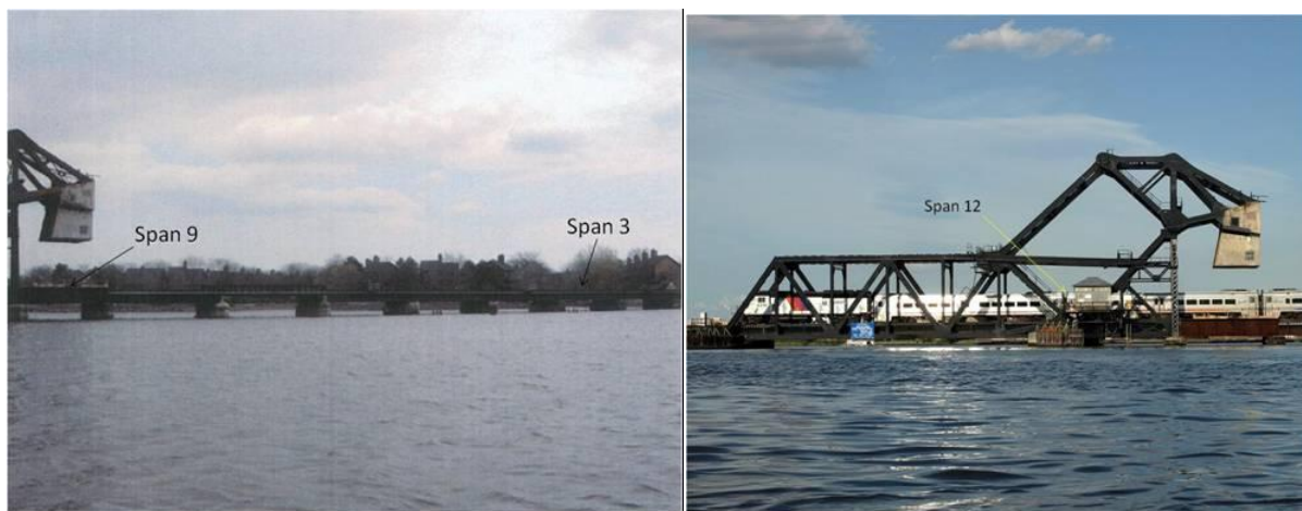
Figure 19. General view of Span 3, Span 9 and Span 12 of the Bergen County Line MP 5.48 (HX Draw) Bridge over Hackensack River Bridge from Inspection Report Cycle 4 (21)
