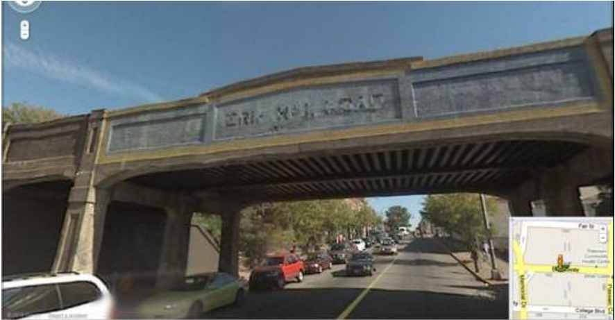
Figure 17. Elevation view of the main span and the controlling member for the load rating (center girder), view from Google Maps
