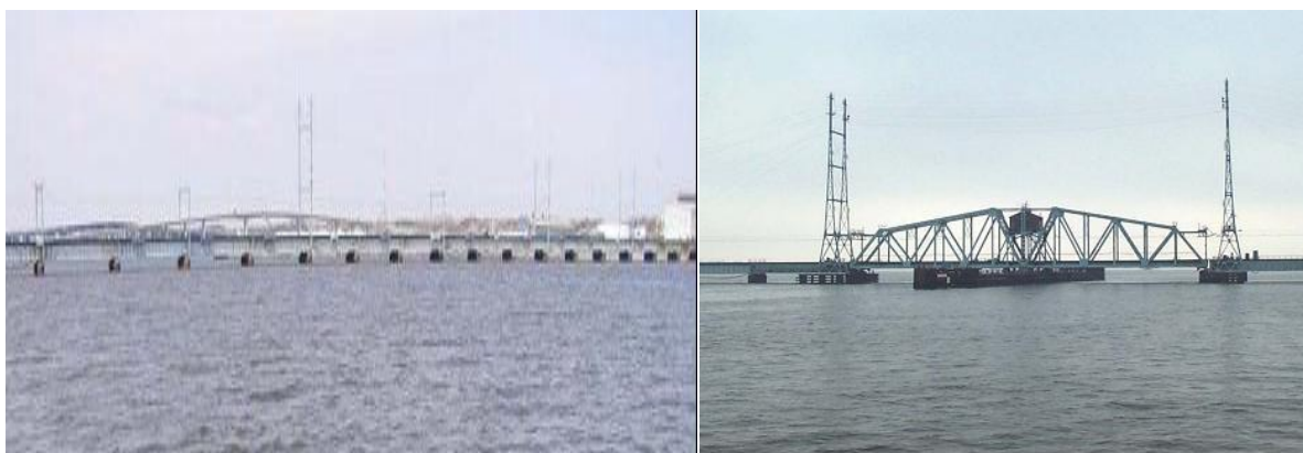
Figure 21. North elevation of east approach Span 1 to 18 of the River Draw Bridge taken from Inspection Report Cycle 4 (23)
