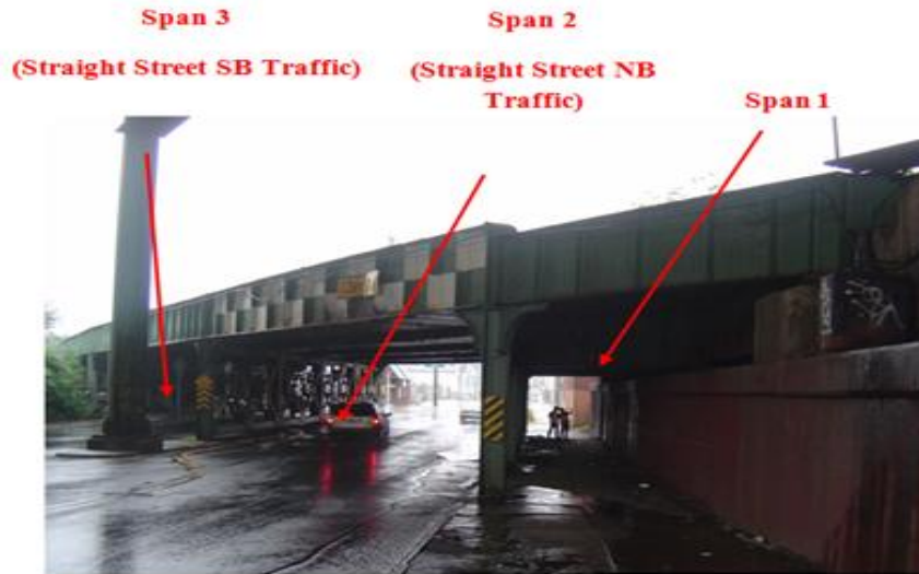
Figure 31. Instrumented Spans 1, 2, and 3 of the Main line MP 15.14 Bridge.
