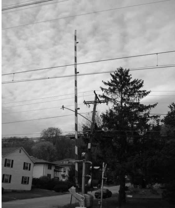
Figure 36. Northern crossing gate
