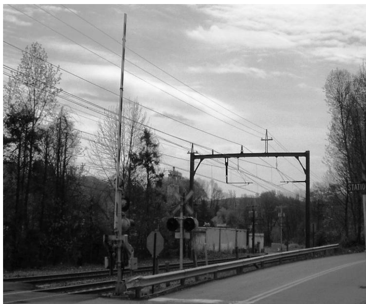
Figure 38. Southern crossing gate and support structure
