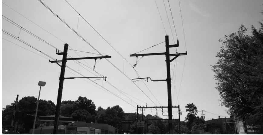
Figure 14. Support structure near Claremont Avenue on the Montclair-Boonton Line
