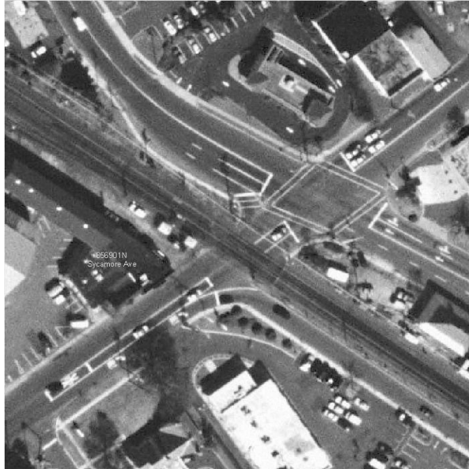
Figure 29. Satellite image of Sycamore Ave crossing
