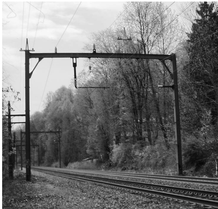
Figure 35. Support structure to the south of Station Rd. crossing
