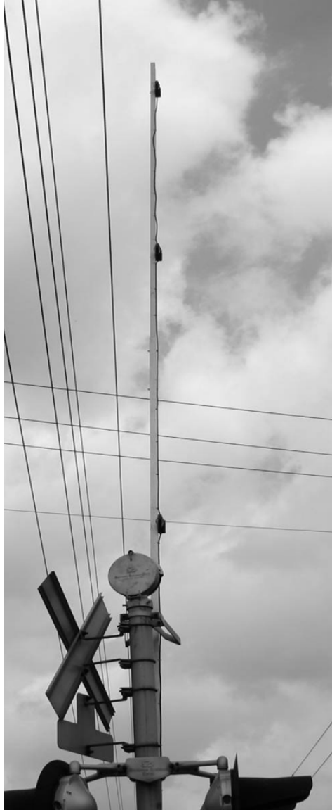
Figure 33. Crossing gate arm at SE corner
