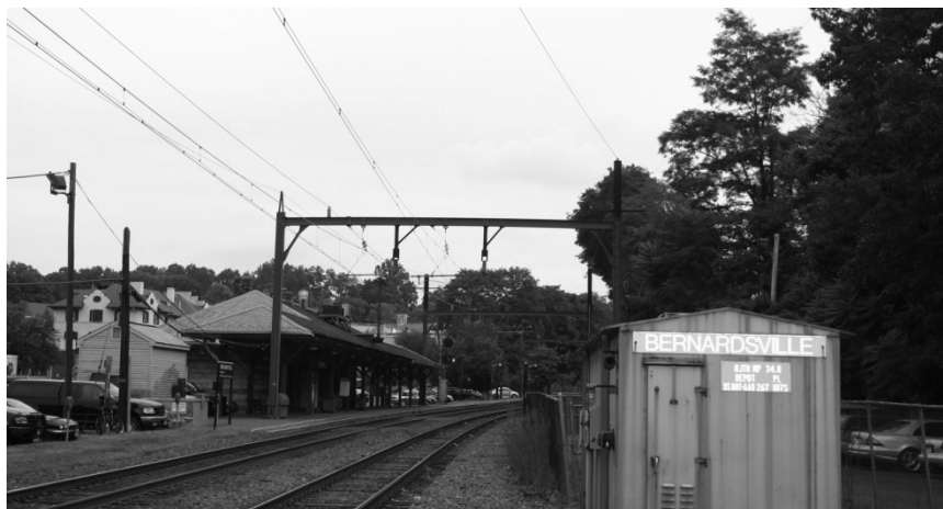
Figure 13. Support structure near Freighthouse Road on the Gladstone Branch
