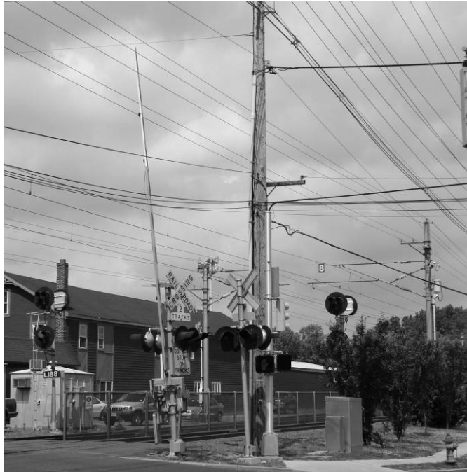
Figure 30. NW crossing gate
