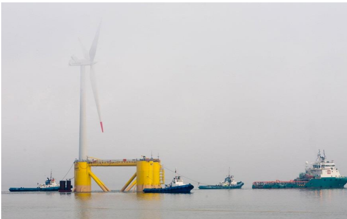
Figure 21. Oceangoing Tugs Towing a Floating Jacket-Mounted Turbine
