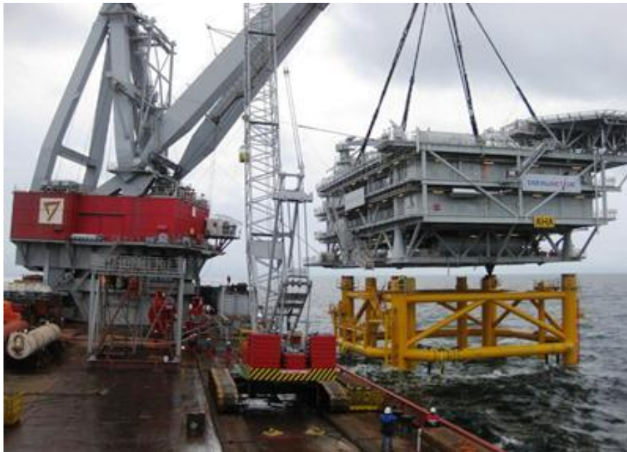
Figure 20. Heavy Lift Vessel Stanislav Yudin During the Installation of an Offshore Substation
