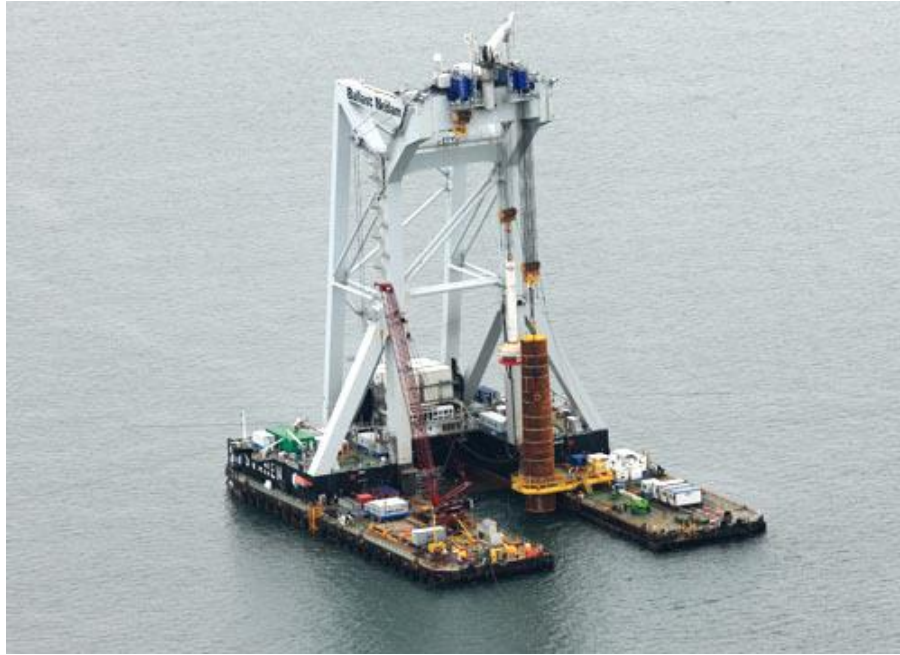
Figure 19. Heavy Lift Vessel Svanen During the Installation Of A Monopile Foundation
