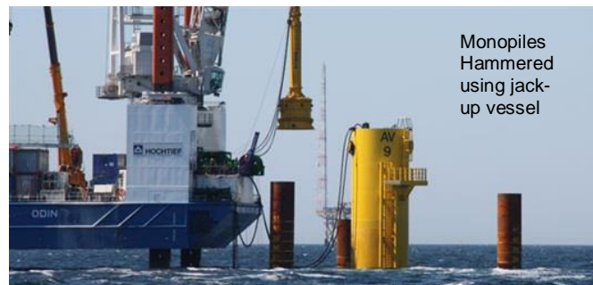
Figure 5. Offshore Wind Farm Installation Process
