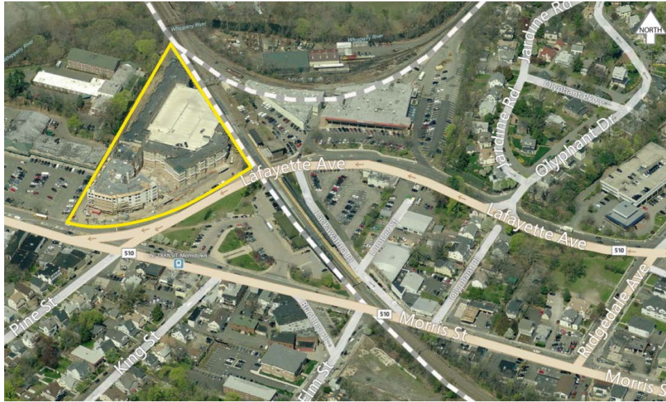
Figure 37. The Highlands at Morristown Station site
