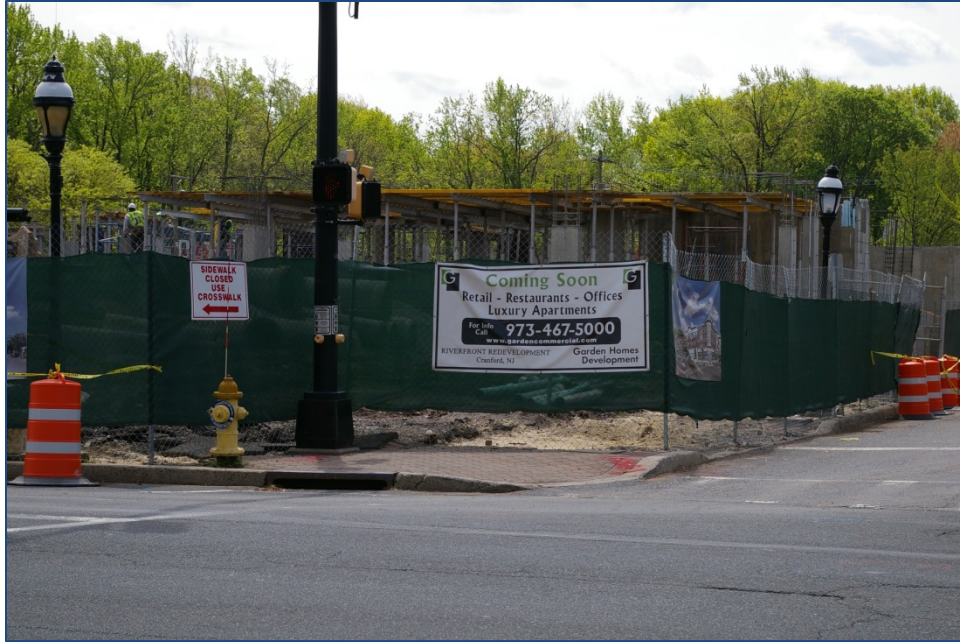
Figure 30. Riverfront at Cranford Station, under construction (Spring 2012)
