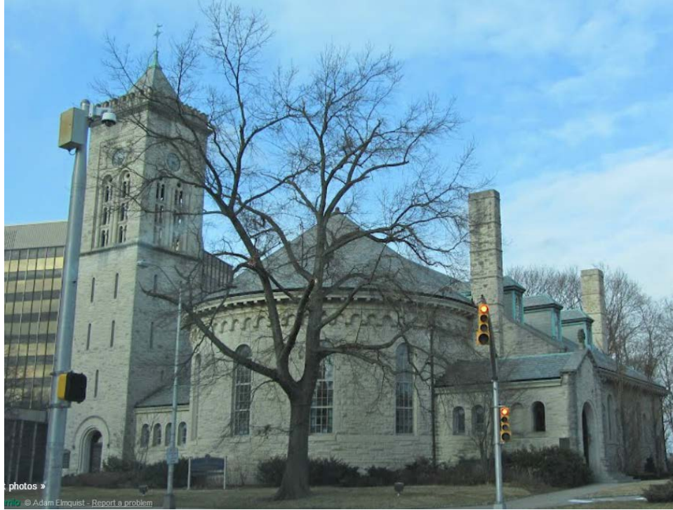
Figure 45. First Presbyterian Church, Morristown, NJ
