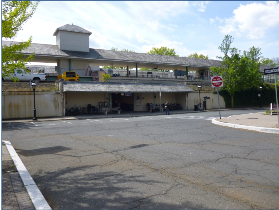
Figure 31. North Ave entrance to Cranford Station (inbound)
