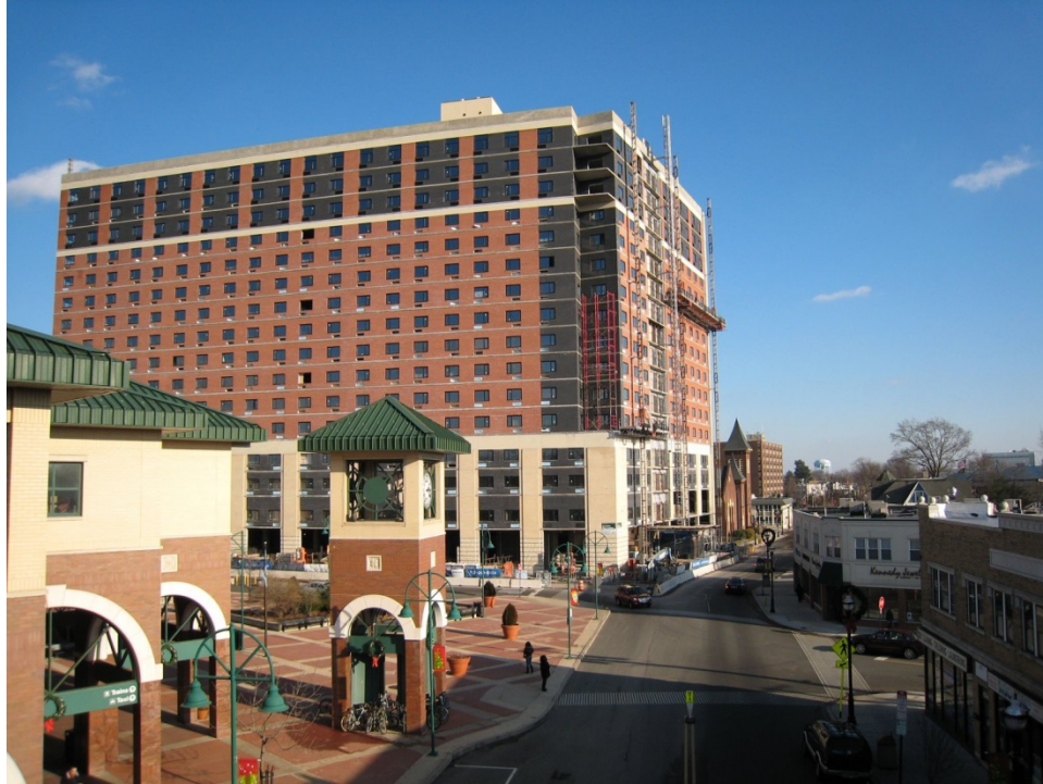
Figure 4. Carriage City Plaza as seen from the Rahway Station platform
