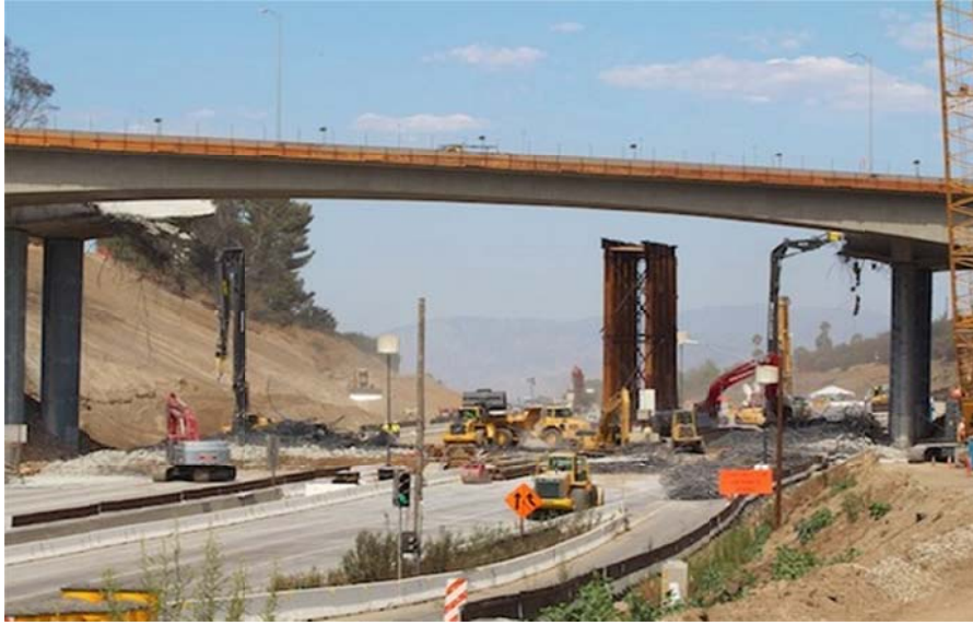
Figure 13. CALTRANS Work Zone Consolidation (Mulholland Drive Bridge) (15)
