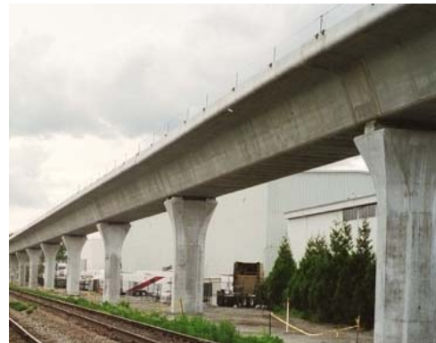
Figure A-21 - Conventional Transit Guideway
