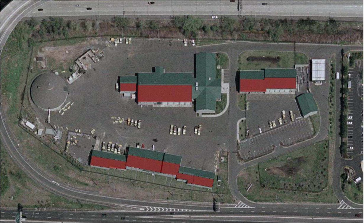
Figure 38. Newark gross roof area
