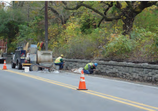
Workers repair historic stone wall.
