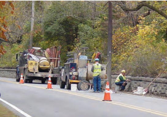
NJDOT workers repair the stone wall along Rt. 29.
