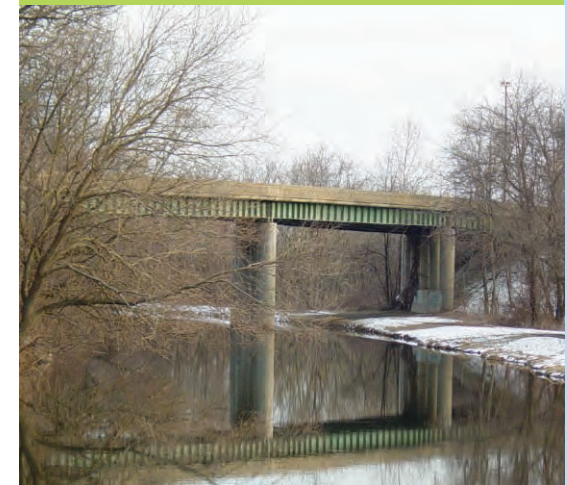
The Scudder Falls Bridge passes over The D&R Canal and multi-use path.
