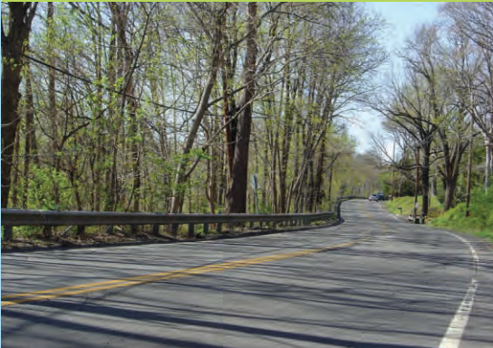
Two lanes from I-95 to Lambertville (MP 18.1)
