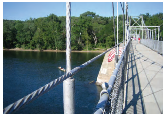
Lumberville-Raven Rock Pedestrian Bridge
