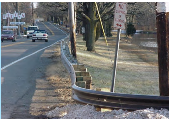
New guiderail along Route 29
