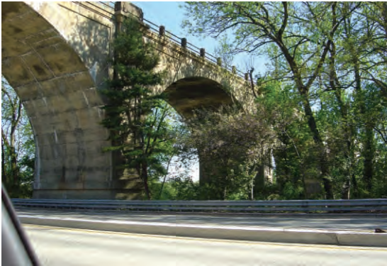
Stone arch railroad bridge – Ewing Township
