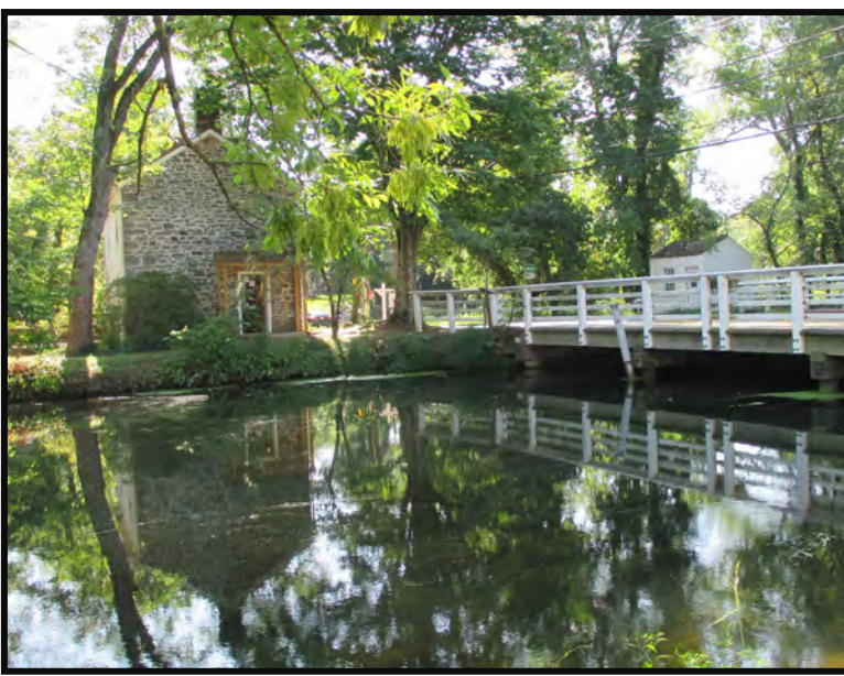
Griggstown Bridge Tender's House
