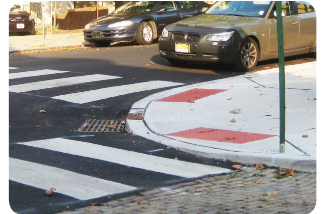
Intersections should have two perpendicular, ADA-compliant curb ramps per corner. Image: The RBA Group
