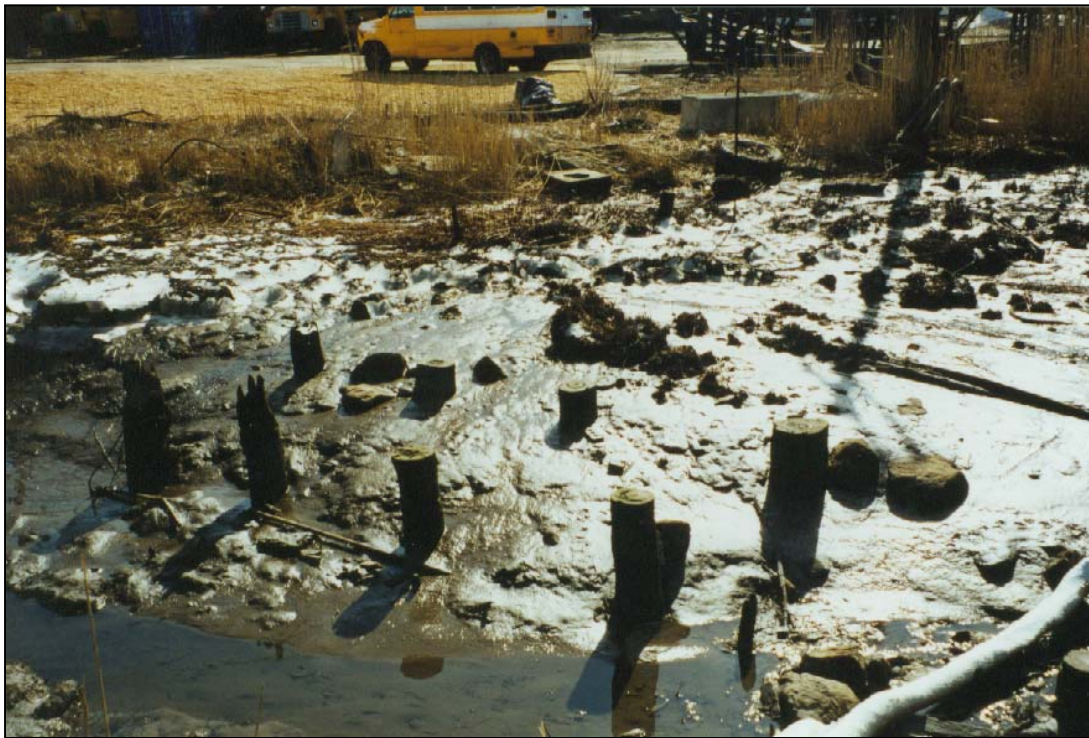
Plate 4.5. Photographs of remains of pilings for the Jersey City Water Works Pipeline at the Hackensack River. A double row of pilings supported the 20" main on cross-beams. Top view is toward the west-southwest, bottom toward the southeast. Photograph: Jean Howson, February, 2001.
