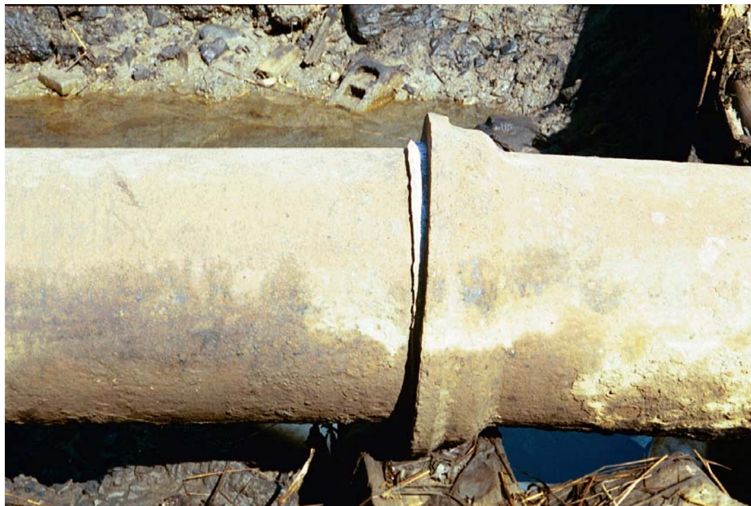
Plate 4.4. Exposed abandoned sections of 20” cast iron water pipe near the Hackensack River. Top: View is toward southwest, with Pulaski Skyway in background. Bottom: View is toward north. Photograph: Jean Howson, February 2001.
