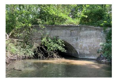
**Proposed project:** NJDOT proposes to fill the undermined area at the north footing with 4.0 cubic yards of concrete and install riprap along the entire length of both the north and south footings at elevation with the creek bed.
