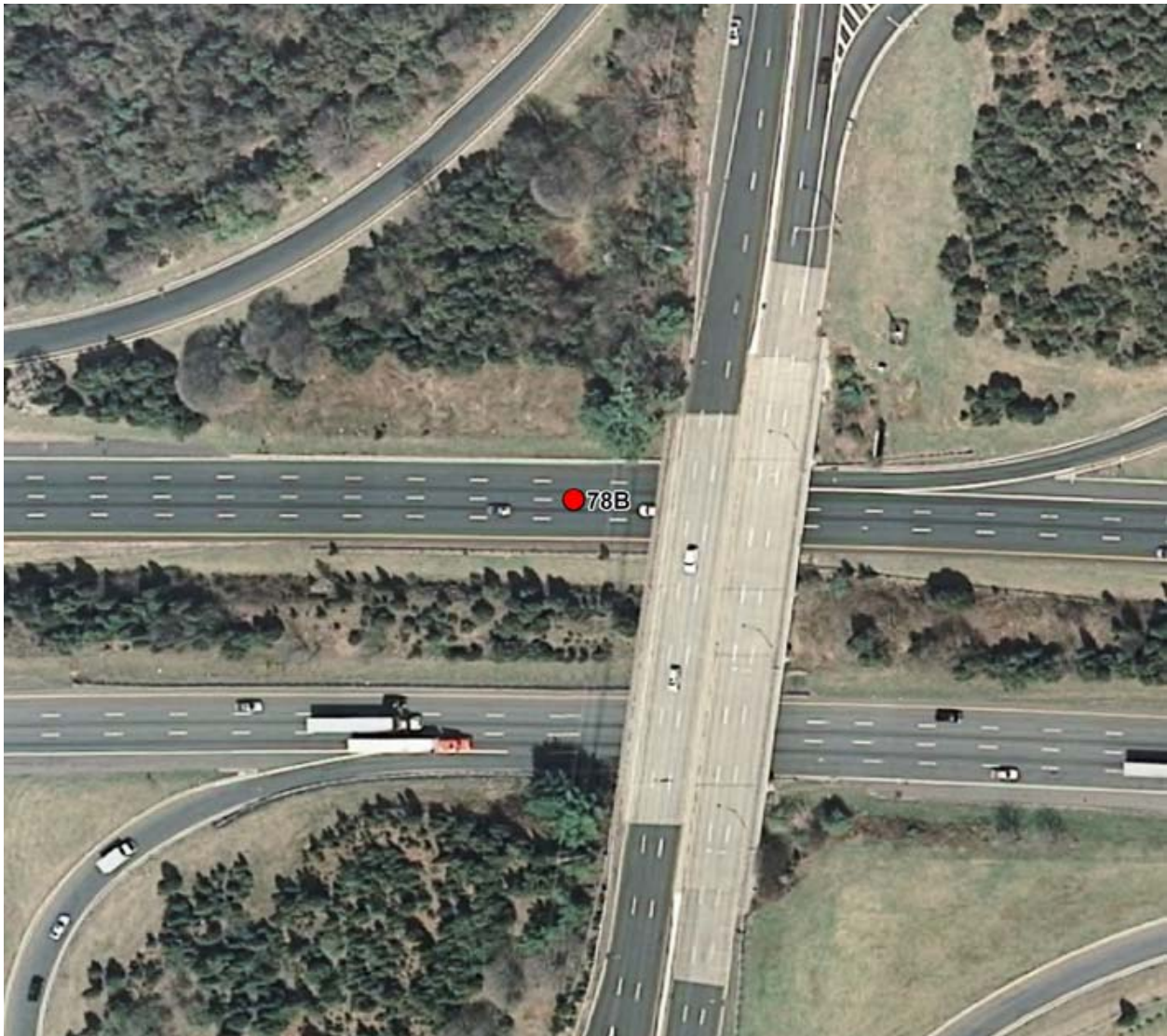
Figure 1-78B: Aerial View of WIM Station at I-78, MP 34.5
