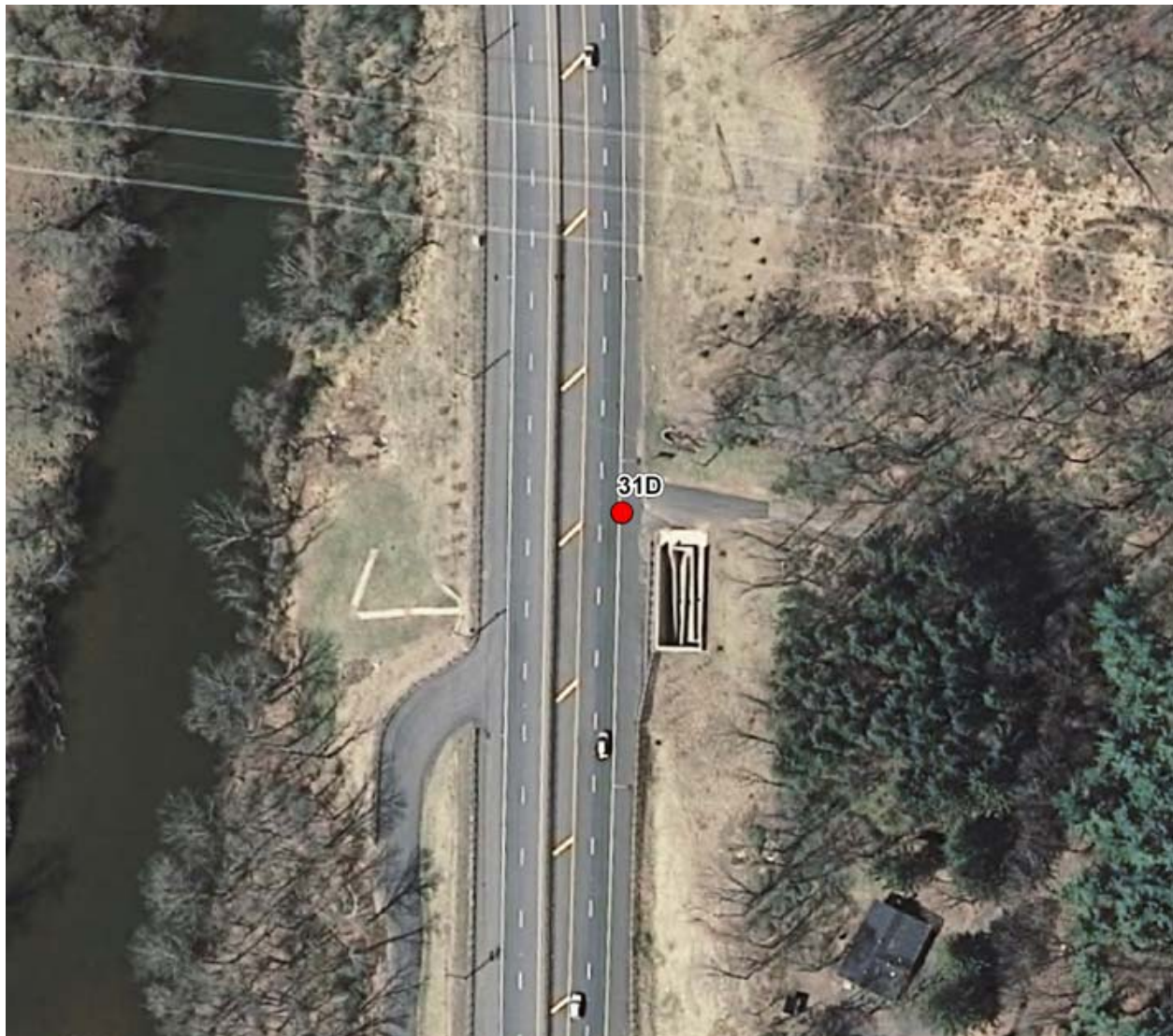
Figure 1-31D: Aerial View of WIM Station at NJ 31, MP 26.4
