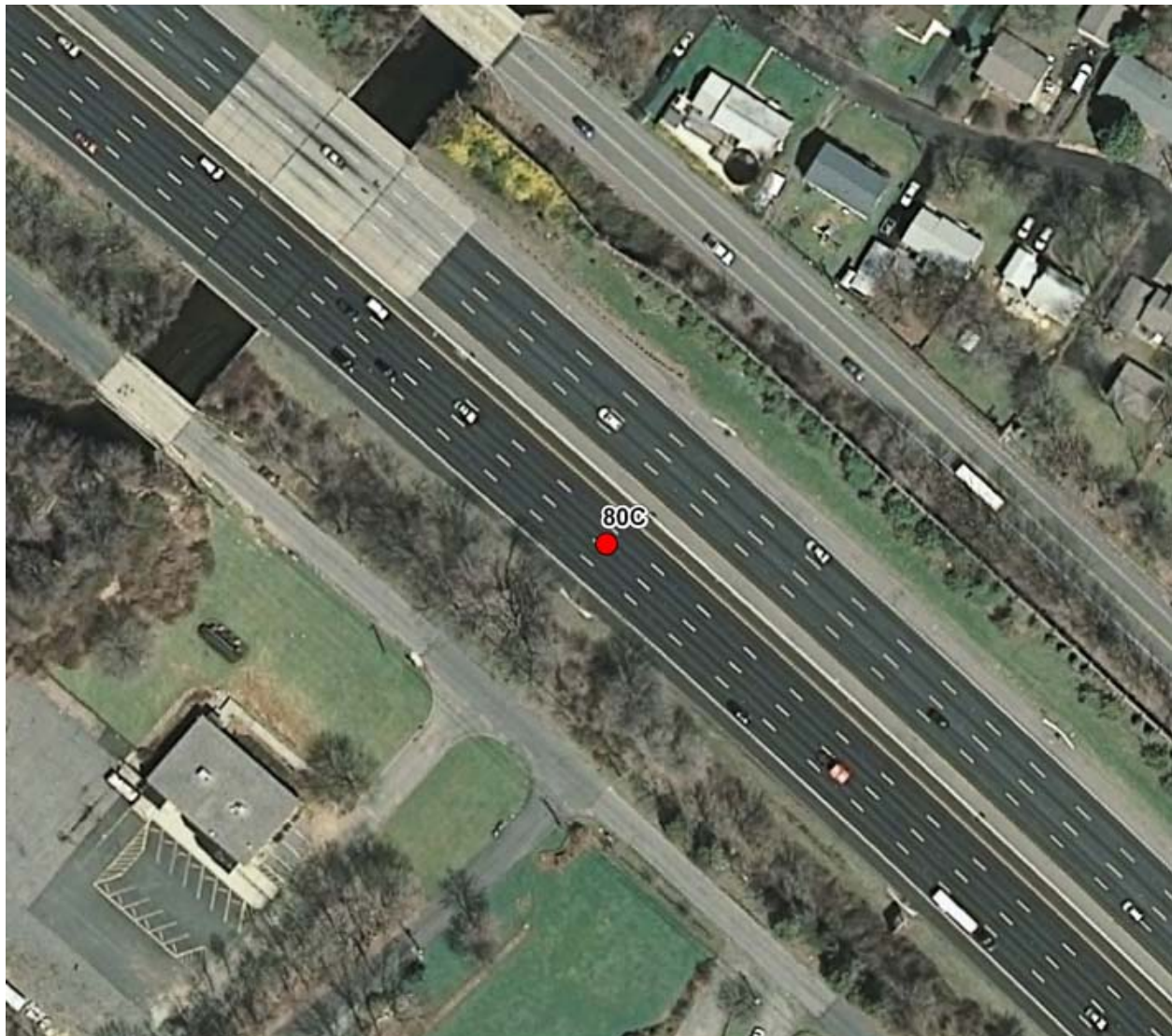
Figure 1-80C: Aerial View of WIM Station at I-80, MP 38.1
