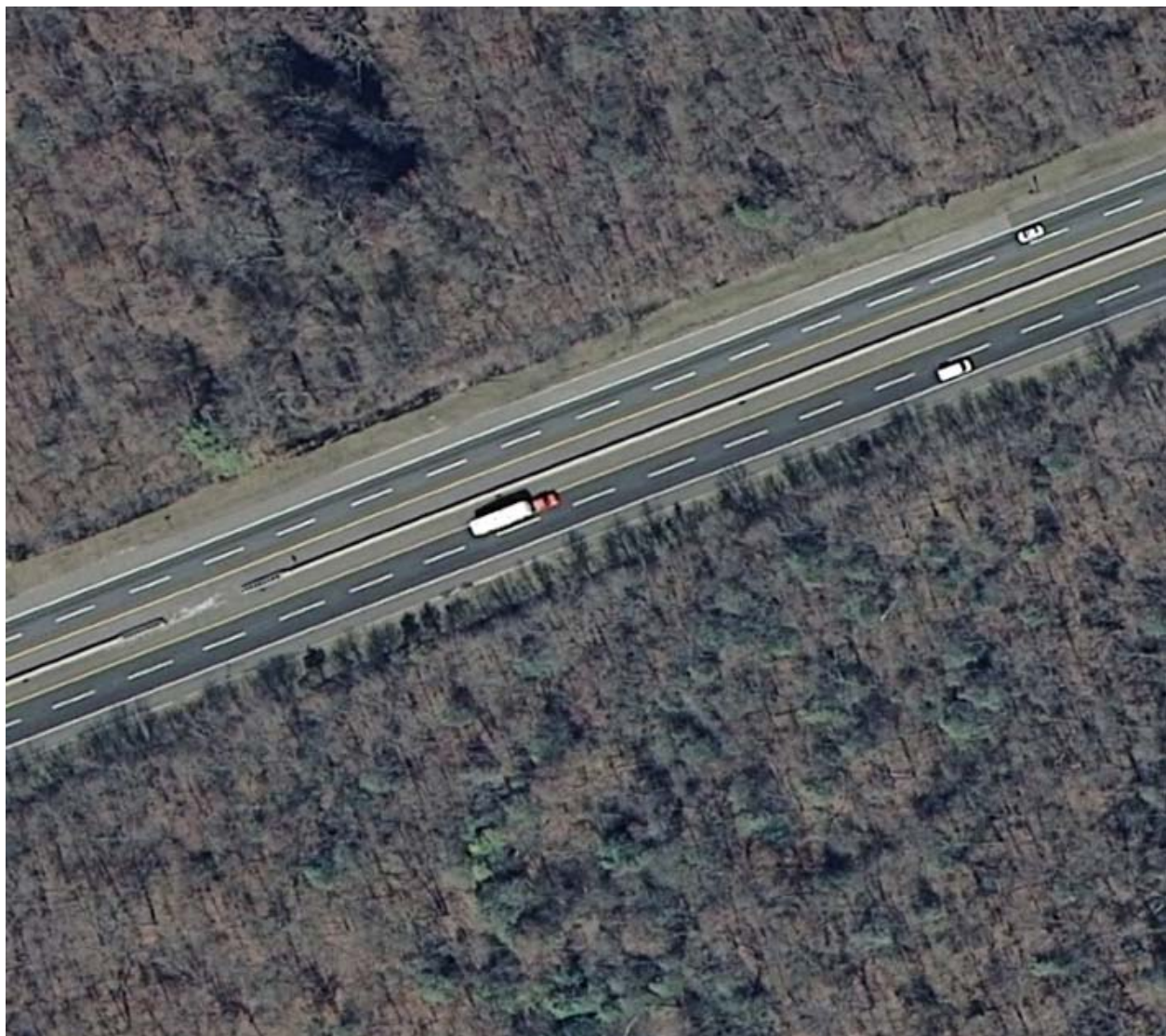
Figure 1-700_1-2: Aerial View of the New Jersey Turnpike Between Interchanges 1 and 2
