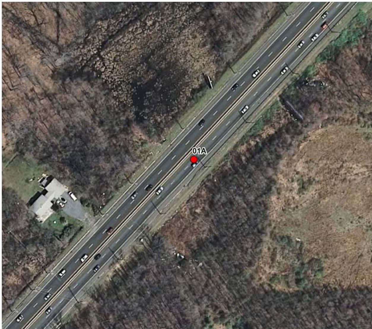
Figure 1-01A: Aerial View of WIM Station at US 1, MP 18.0
