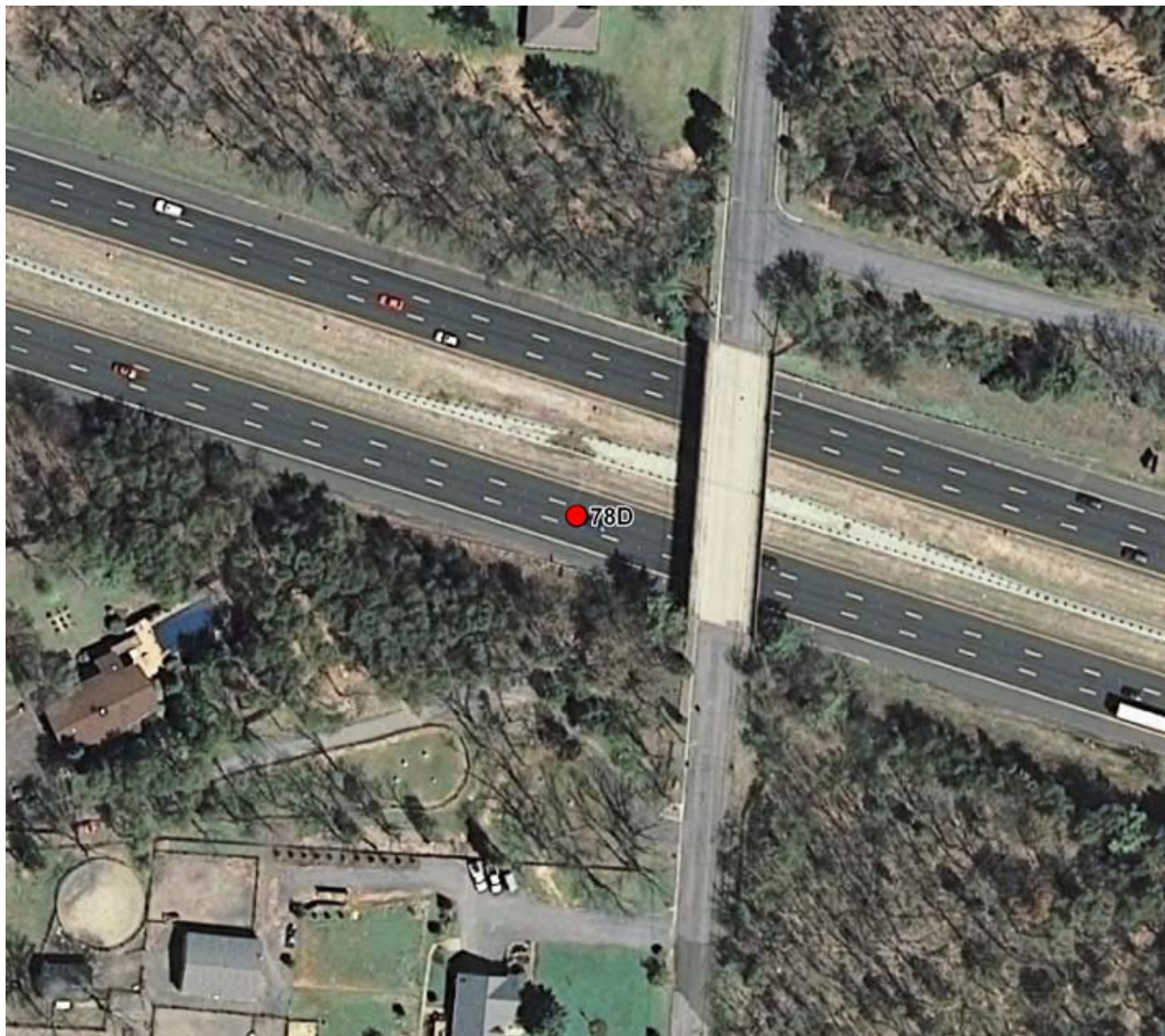
Figure 1-78D: Aerial View of WIM Station at I-78, MP 25.7
