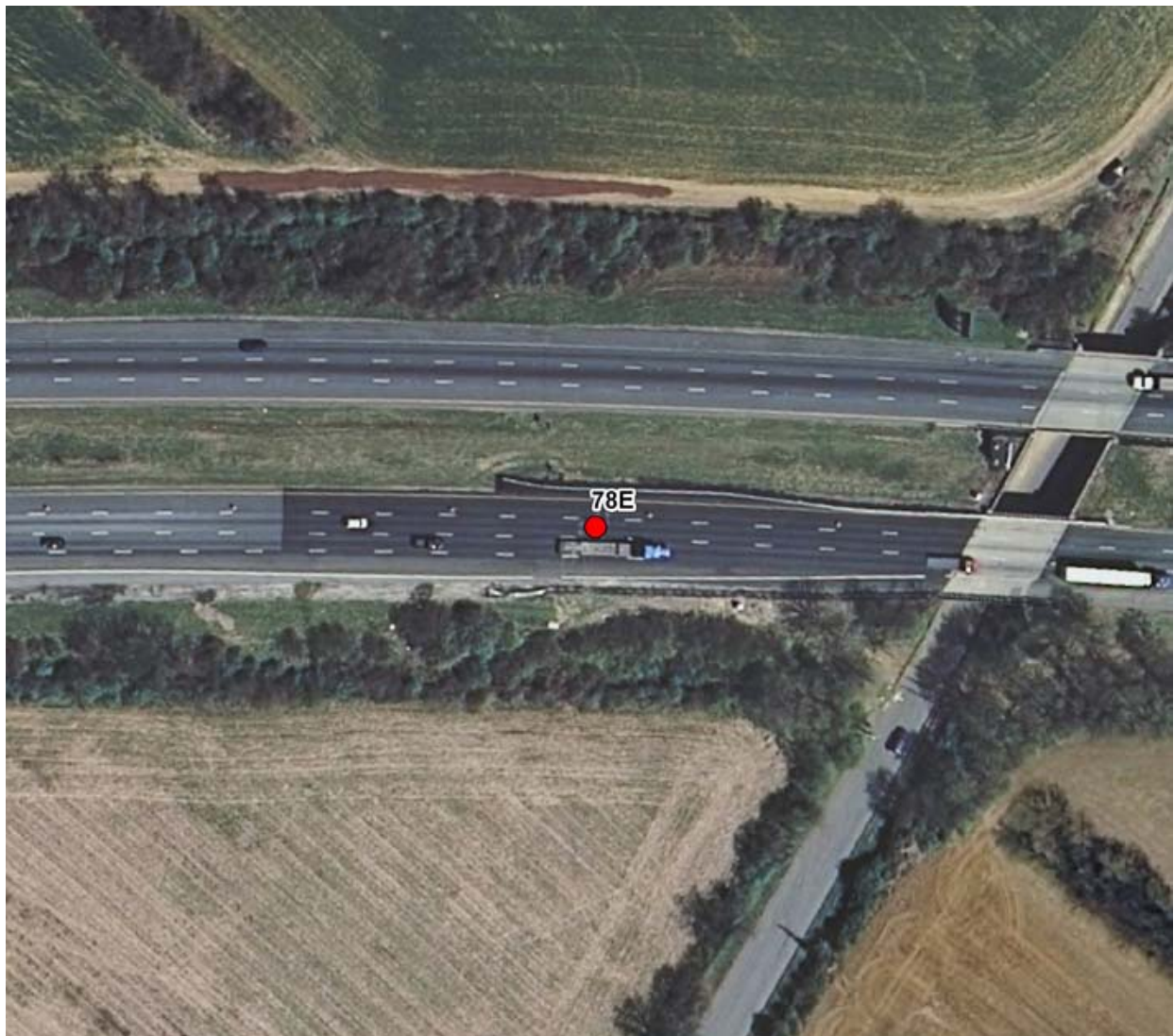
Figure 1-78E: Aerial View of WIM Station at I-78, MP 5.02
