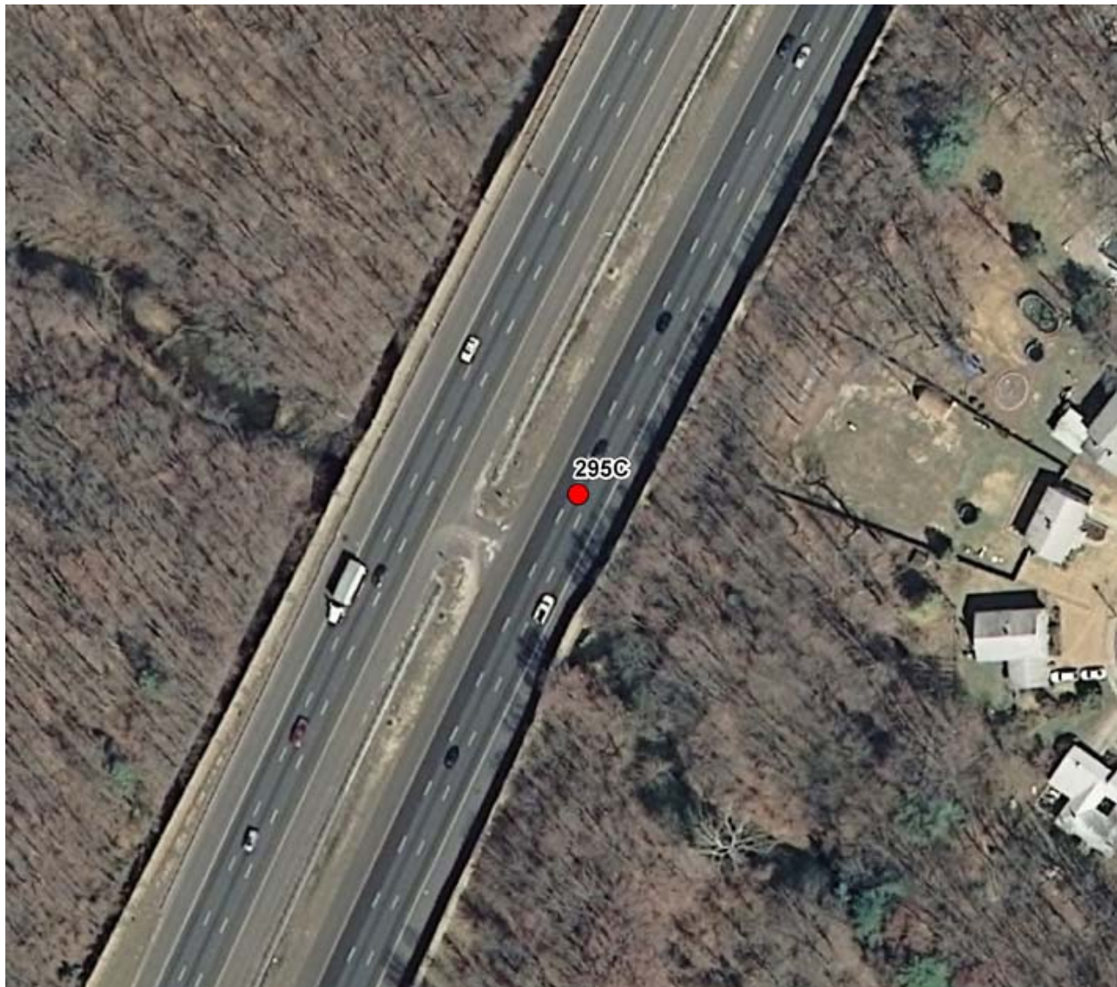
Figure 1-295C: Aerial View of WIM Station at I-295, MP 35.7
