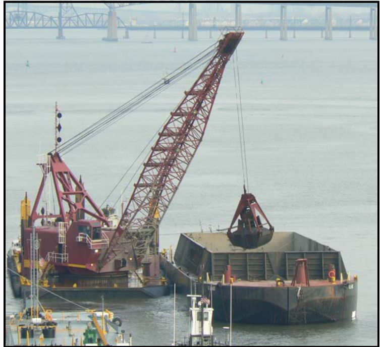
The Great Lakes Dredge #54 as it works to dredge in the Newark Bay. Photo courtesy of the Sandy Hook Pilots Association.
