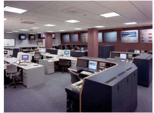
Verizon 9-1-1 Control Center in Piscataway just prior to going in service in 1998.
